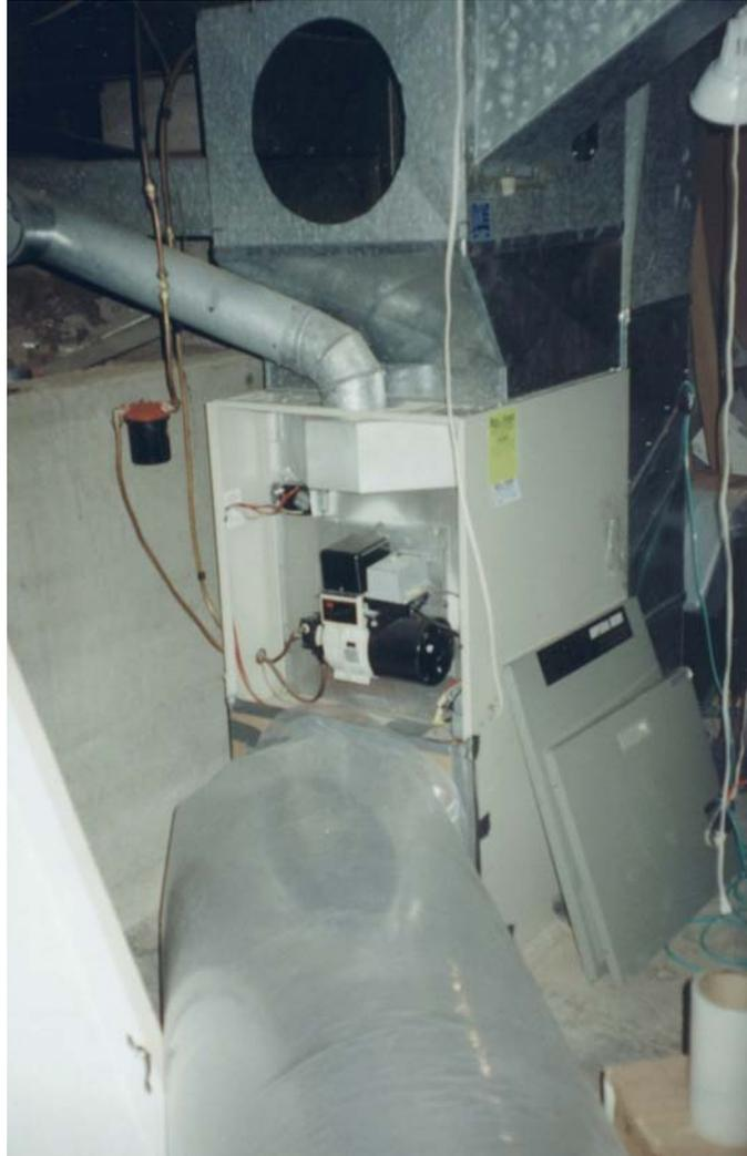
**Fig. 2.2. The Aeroseal tubing connection.**
