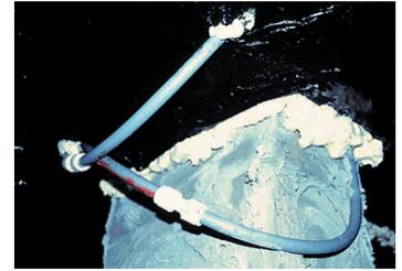
Bottom board penetrations sealed with patch and foam
