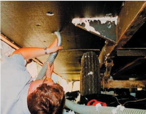
Blowing insulation into the floor cavity
