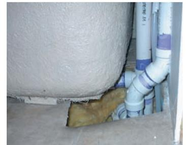
Hole in floor at plumbing penetration behind tub
