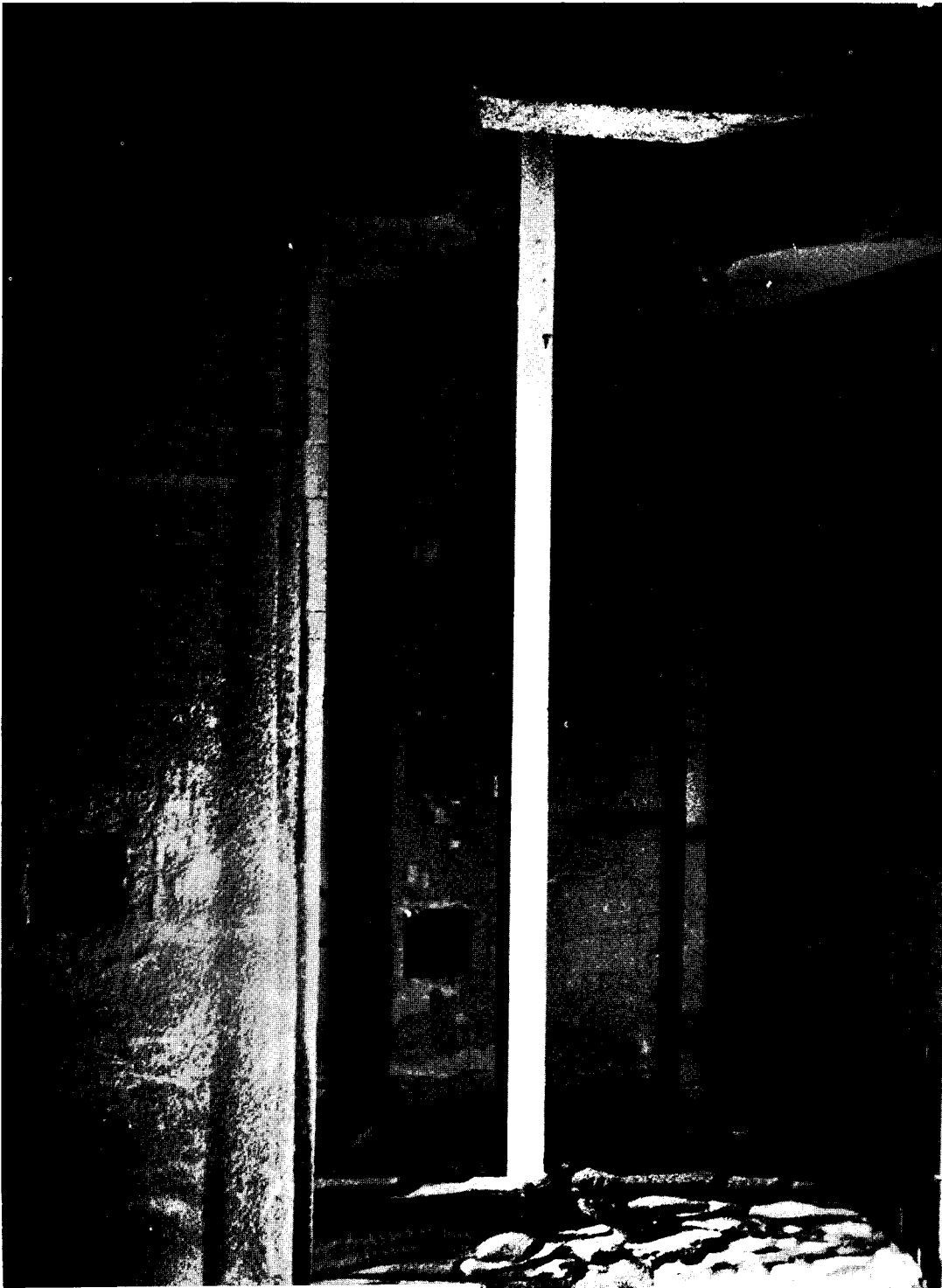
Figure 1. The column assembly in place prior to fire test.
