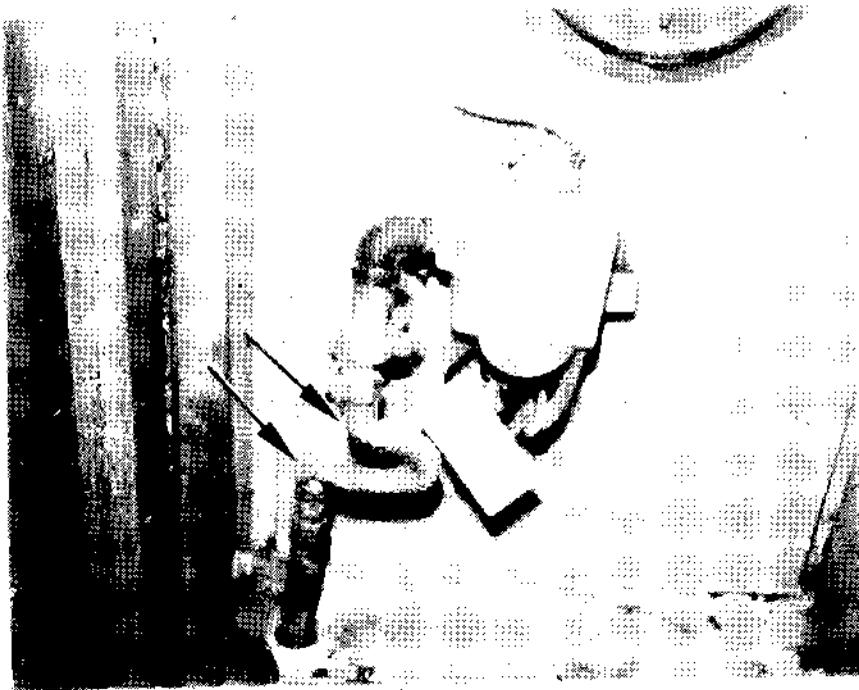
Figure C-84 Flexible Gas Connector on Furnace
