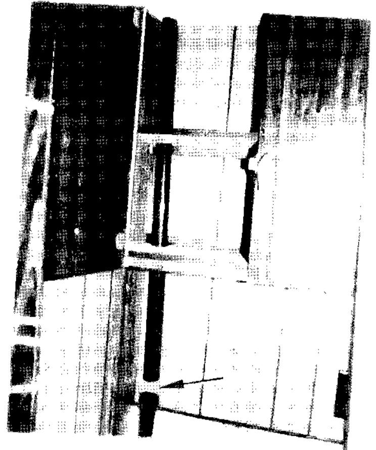
Figure C-71 Plastic Drain Pipe Fitting Has Not Been Properly Adhered with Adhesive.
