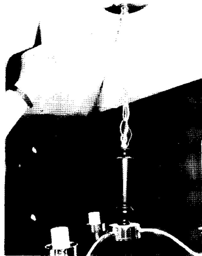
Figure C-105 Grounded Pendant Fixture.
