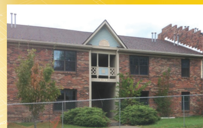
Centre Meadows (Lexington, KY before RAD construction)
