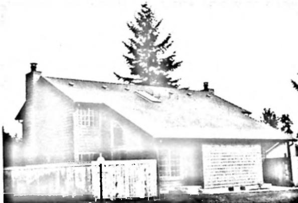
The smallest loft home contained 648 square feet and the largest, 674 square feet. The main level consisted of a living room with a vaulted ceiling, a dining area with vaulted-open beam ceiling and a kitchen. The upper loft area contained one bedroom and a bath.
