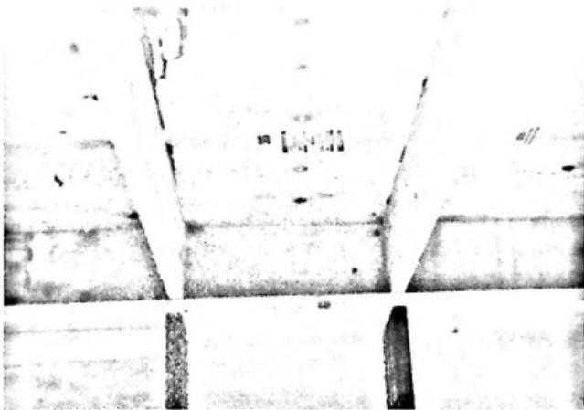
require bridging only in floors with joists exceeding a depth-to-thickness ratio of 6 to 1 based on nominal dimensions. In other words, joists up to and including 2x12s do not require mid-span bridging.
