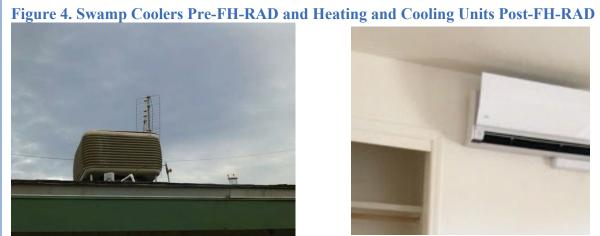
Swamp coolers (on the left, provided by FH) were replaced with the wall-mounted heating and cooling (mini-split) units, which were installed in each room.
