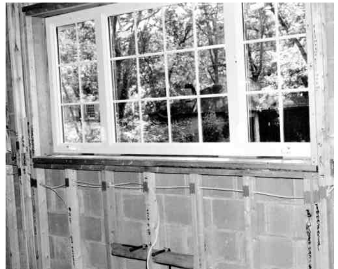
Figure 6-6: Plumbing Rough-In on Exterior CMU Wall
