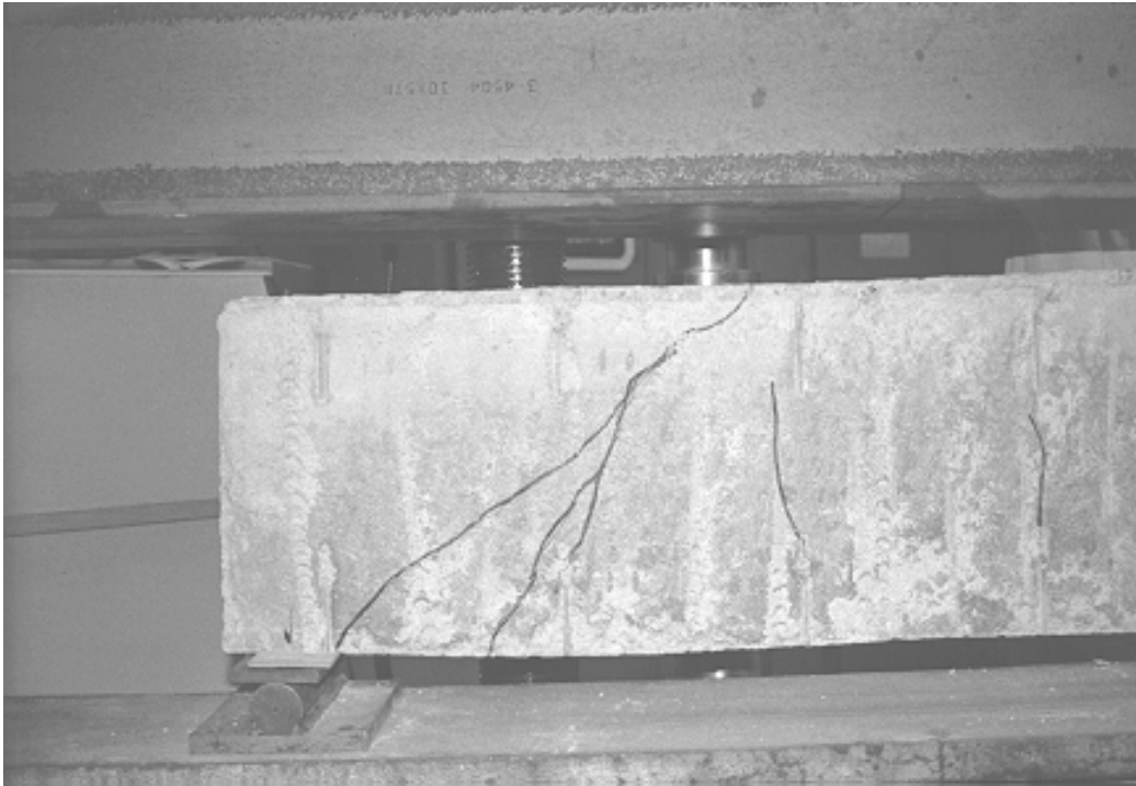
Figure 6 Typical Failure Mode for the ICF Flat Lintel
