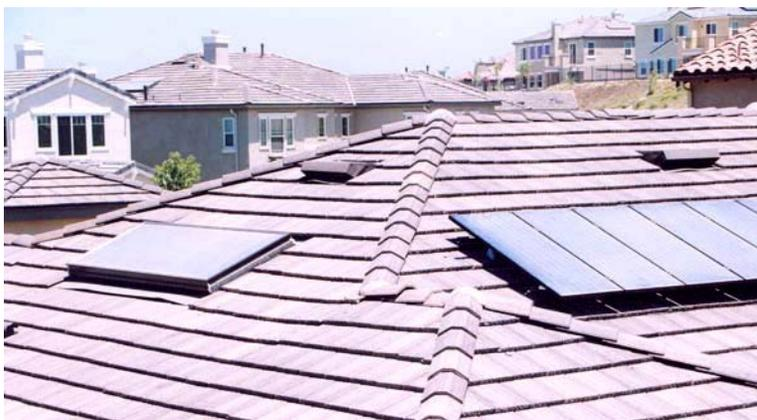
Figure 4 – Low profile solar pre-heat of domestic water (on left of roof) at PATH field evaluation in San Diego (source: Toolbase)
