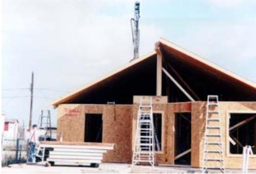
Figure 5 - Roof panels at PATH field evaluation in Texas
