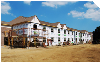
Hudson Companies' first LEED Project under construction in North East, PA.
