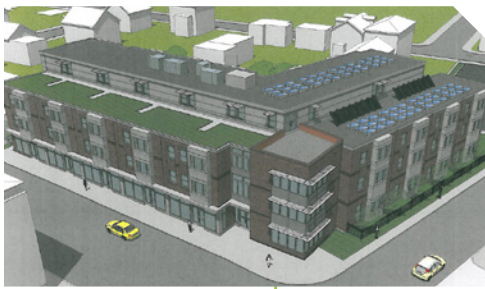
Rendering of Quincy Commons showing green roof and solar panel elements.
