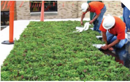
Quincy Commons will have a green roof by LiveRoof ( www.liveroof.com ) which eliminates air gaps between modules to prevent warm or cool air from escaping from the building below.
