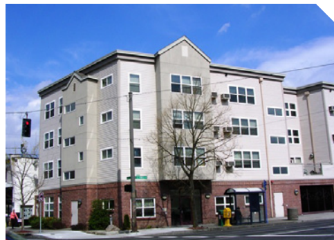
Green Retrofits underway at Powell Boulevard Apartments.
