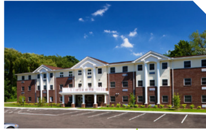
Construction completed in Garden Way Apartments.
