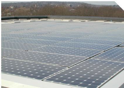
Solar array on a Section 202 property in Somerville, MA.
