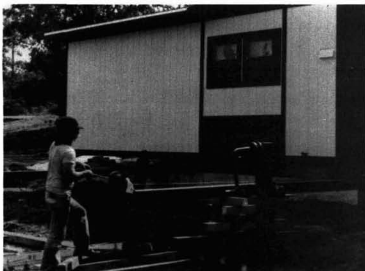
Brinkley-winch system of placing unit on foundation
