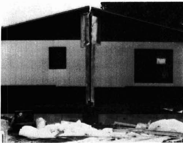
Two sections being joined on site to form a double-wide unit
