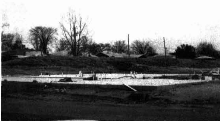
Slab-on grade foundation
