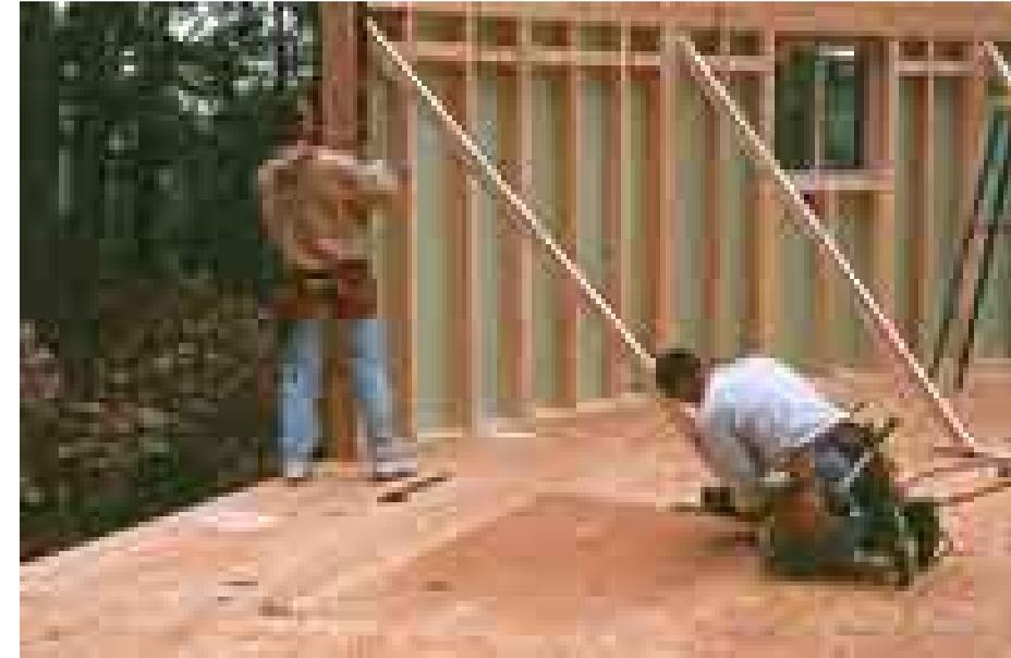
*Wood-based open-wall system is the closest technology to conventional stick framing*
