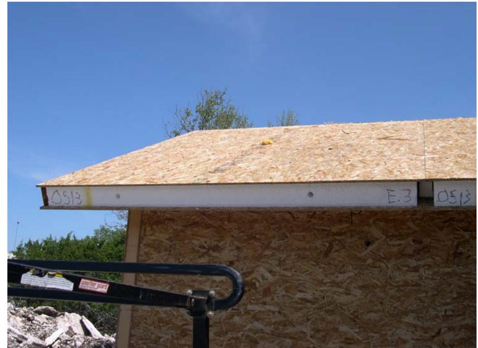
*Structural insulated panels are used for roofs as well as walls, with pre-cut channels*
