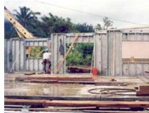
*Open-wall system allows access for utilities*
