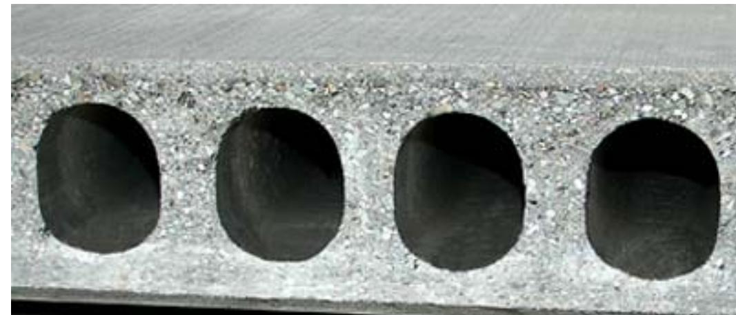
*Concrete panel core is hollow for utility chases and to lighten the members*
