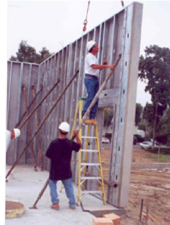
*Concrete panels have open-wall of steel studs*
