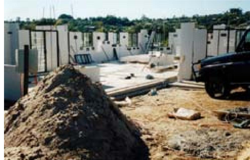
*Erection on-site of AAC concrete panels*
