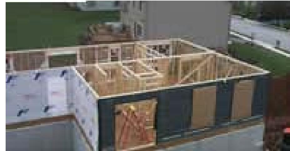
*Exterior open wall panels with stick-built interior partitions*
