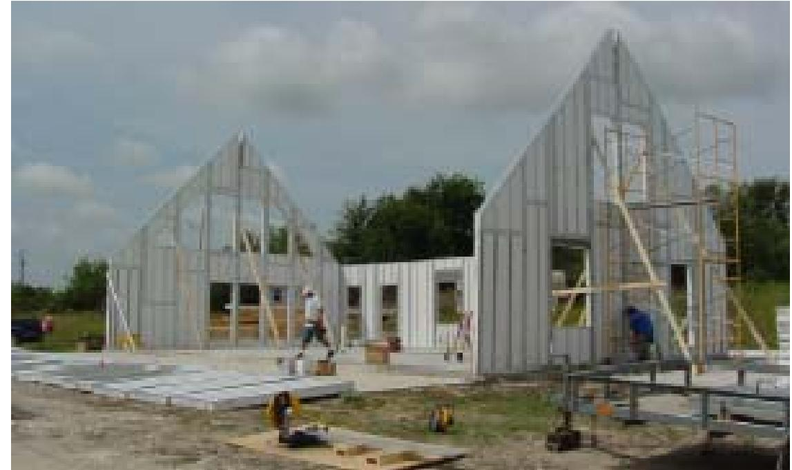
*Metal-skin panels with insulating cores provide superior energy performance*
