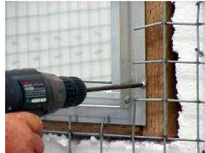
*Wire mesh and insulation is trimmed around window and door openings*
