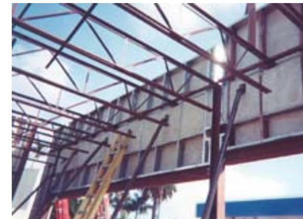
*Roof structure frames into concrete panels*
