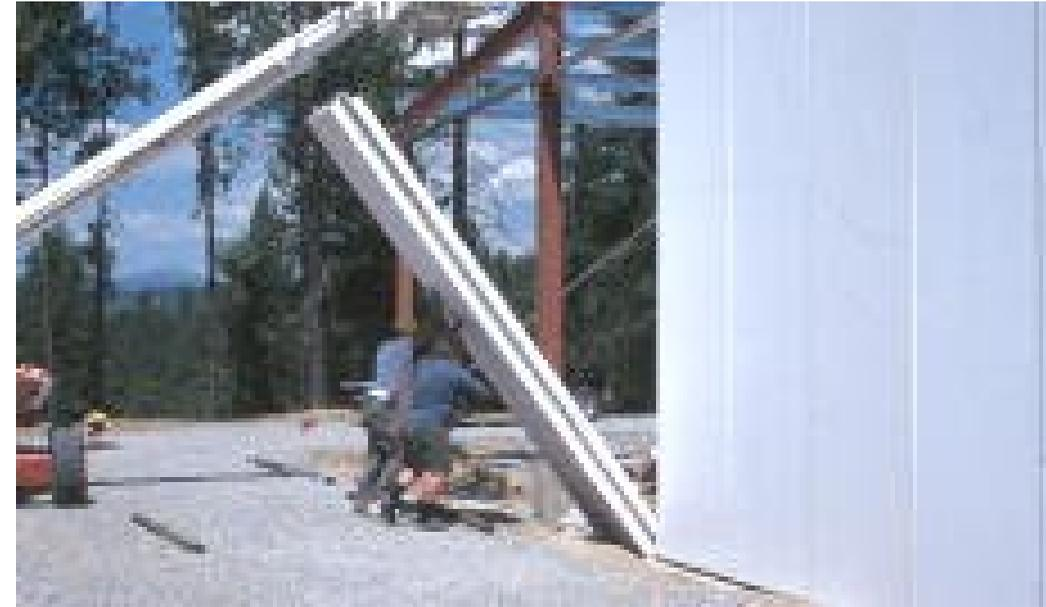
*Steel and foam panels are lighter and easier to assemble*
