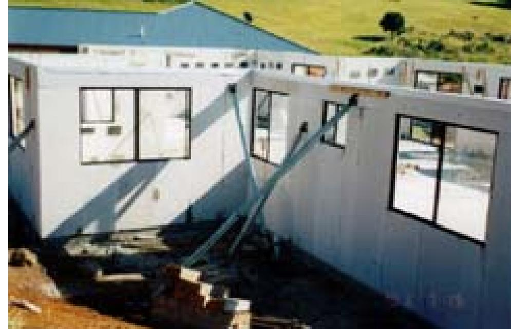
*Panels are stabilized by struts during erection process*
