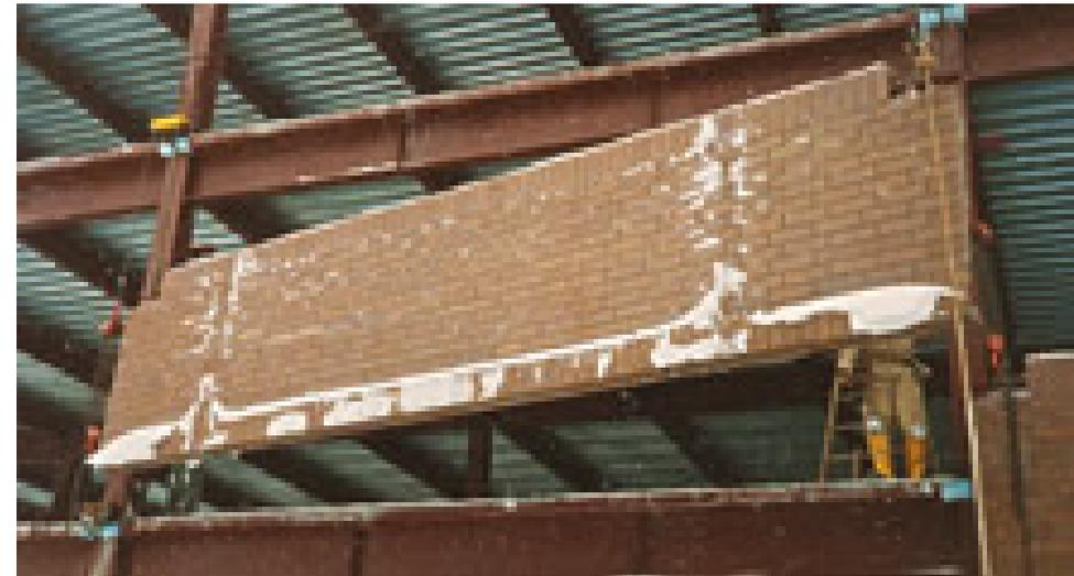
*Panel exterior is finished with brick-and-mortar*
