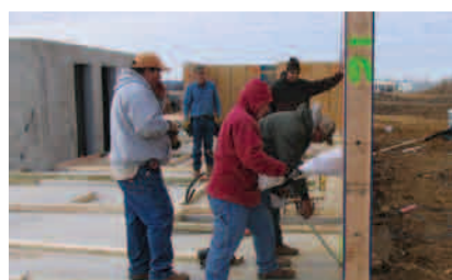
Workers installing SIP walls
