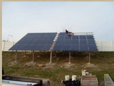
Installation of PV System
