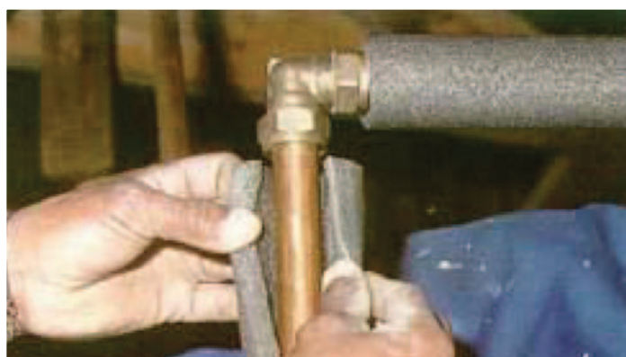
Energy saving pipe insulation
