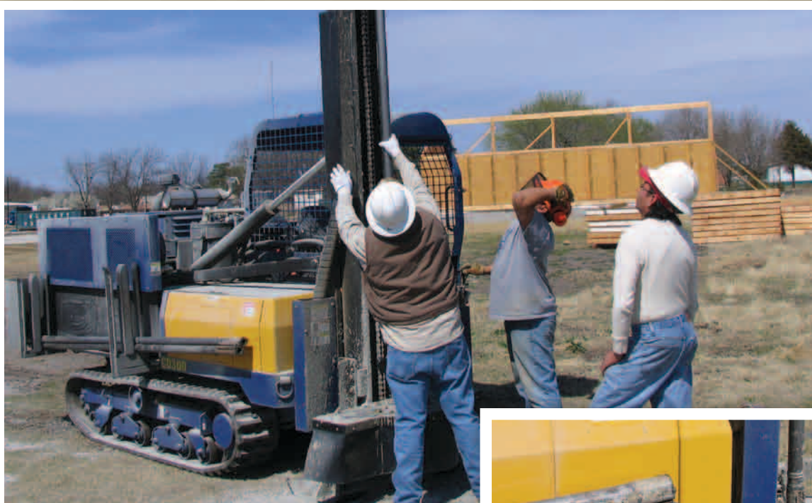
Workers using geothermal drilling rig
