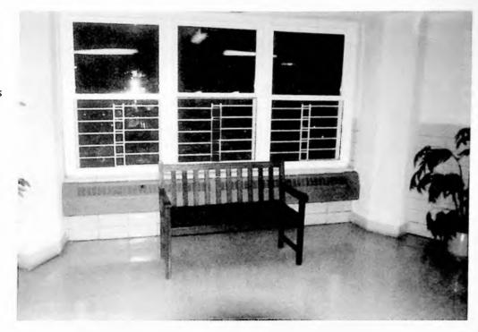
The interior hallway is well lit. Existing glazed block was cleaned for reuse because of its durability and easy maintainability. Lead-based paint on hallway walls was encapsulated with a product which leaves a stucco-like finish on the walls.
