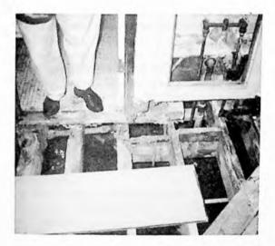
Rot and water damage to floor joists and wall on ground floor.
