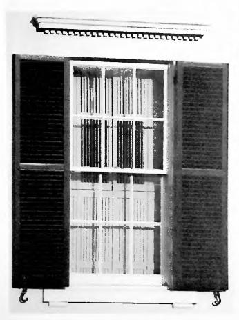
House, District of Columbia (late 19th century). These shutters have fixed lowers, designed more for filtering the sun than for reducing heat loss. Notice the hardware for holding the shutters open so that they do not swing freely. The interior shutters have adjustable vertical slats.
