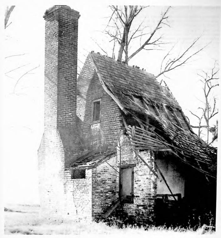
Towles House, Virginia (early 18th century) The chinney placement minimizes the transfer of heat to the interior of the house by reducing the contact area of the chinney mass with the house. The flue is freestanding, reducing not only the heat gain, but the fire huzard as well. The house is no longer standing
