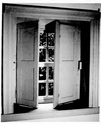
Stratford Hall, Virginia (ca. 1730). Interior shutters, as opposed to exterior shutters, are designed to be invisible when open. Unfortunately, they are frequently stuck in the open position by accumulated layers of paint. This same window is illustrated with the shutters open in the section on splayed window reveals.
