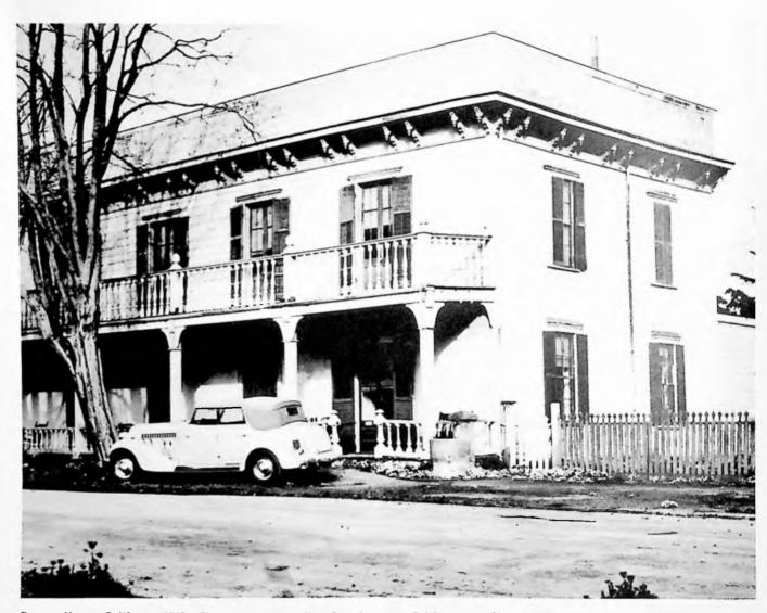
Zanetta House, California (1815). The whitewashed walls reflect the strong California sun. Shutters with movable louvers control the amount of sun passing through the windows. Another feature not readily apparent is that the walls are adobe under the wood sheathing. Adobe has characteristics similar to masonry, thus helping to moderate interior air temperatures.
