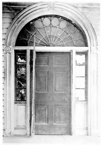
Boykin Hall, Georgia (early 19th century). In addition to providing illumination, the fanlight and side lights are incorporated into an architectural feature that is designed to draw attention to the doorway. Some side lights can be opened for ventilation.
