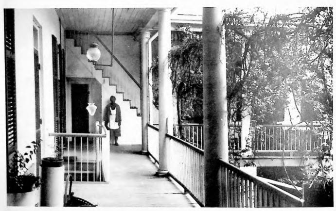
Umbria, Alabama (ca. 1829-30). The two story porch wraps around a courtyard. It not only shades the house but also provides sheltered exterior circulation, appropriate for a warm climate. Shutters with movable louvers and screen doors allow additional control of light and ventilation.
