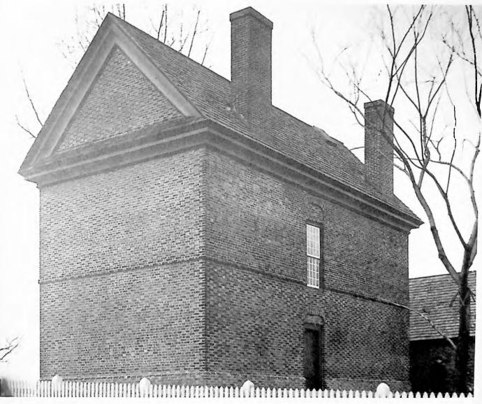
Bel Air (Singley House), Pennsylvania (ca. 1725). The north elevation of this house has no windows except for one which lights the stair landing. There are two interior chimneys in the north wall with fireplaces flanked by closets in each room. The coldest wall in the house is thus isolated from the inhabitants. The closets also serve as warm air convection flues to provide additional heat.
