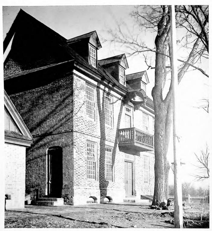
Bel Air (Singley House), Pennsylvania (ca. 1725). The south elevation has three dormer windows, eight large windows with interior shutters, and four basement openings. The doors have transoms that light the center hall on each floor with the middle dormer providing light into the stairwell. Deciduous trees shade the elevation from the summer sun, preventing unwanted heat gain.
