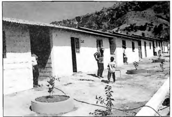
New housing construction in Chiapas, Mexico
