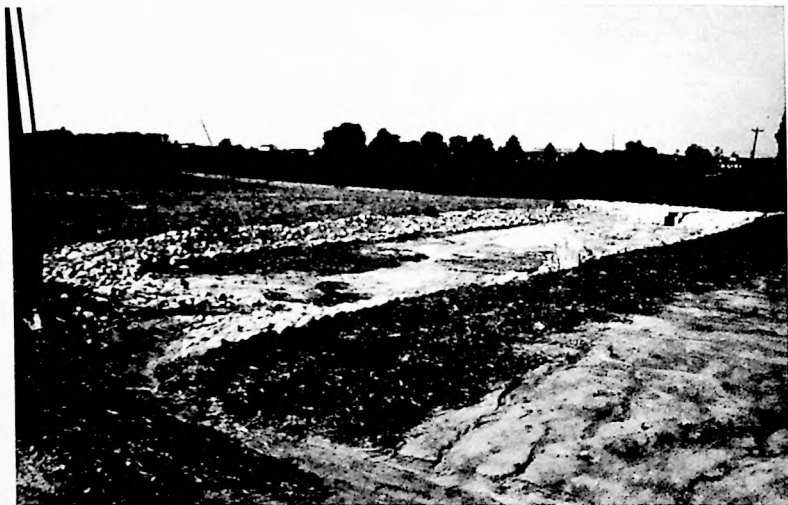
Storm water detention basin
