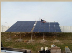
Installation of PV System
