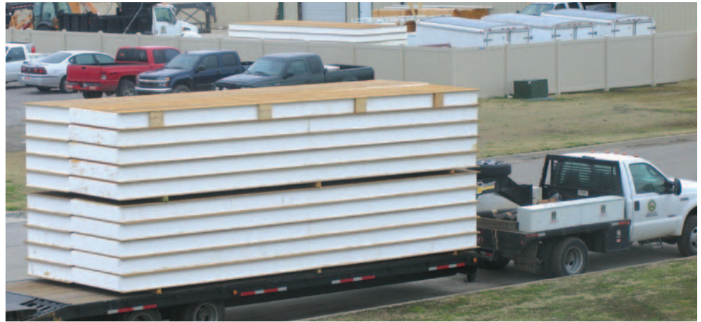
SIPs being transported.
