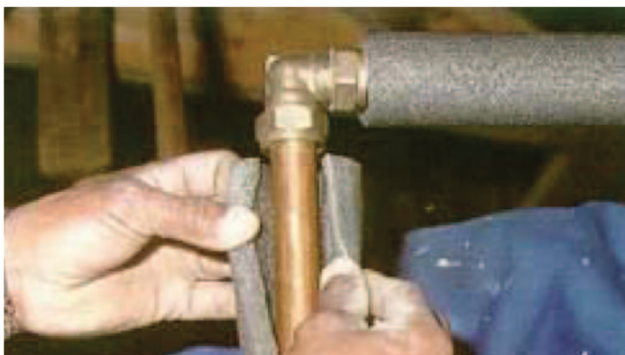
Energy saving pipe insulation
