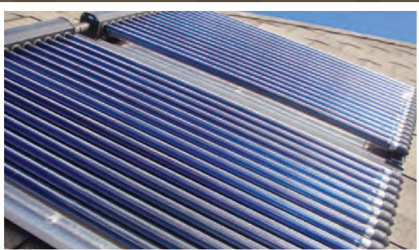
Solar domestic hot water
