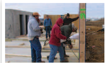
Workers installing SIP walls
