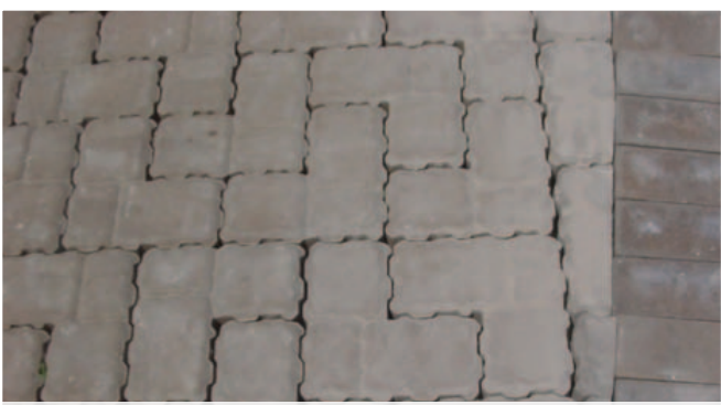
Interlocking permeable pavers
