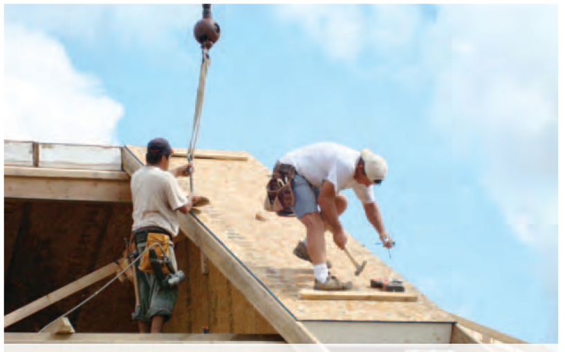
A crane lowers the SIPs roof into place (not at Nez Perce Tribe).
