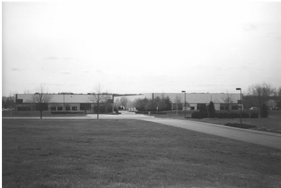
Figure A-23 - View Looking West (Station 4)
