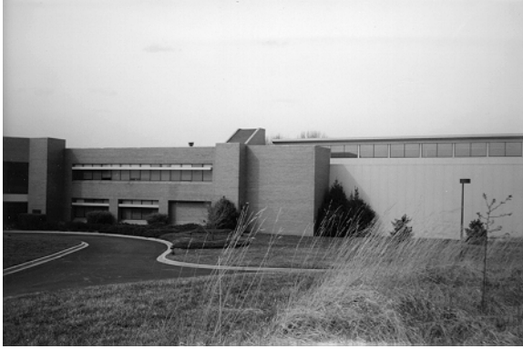
Figure A-17 - View Looking North (Station 4)
