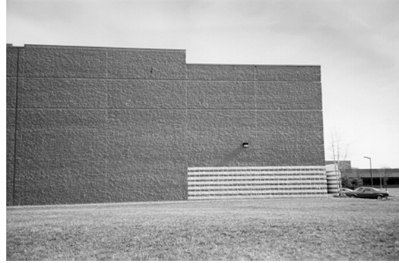
Figure A-34 - View Looking Northeast (Station 6)
