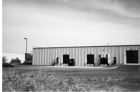
Figure A-10 - View Looking Northeast (Station 3)
