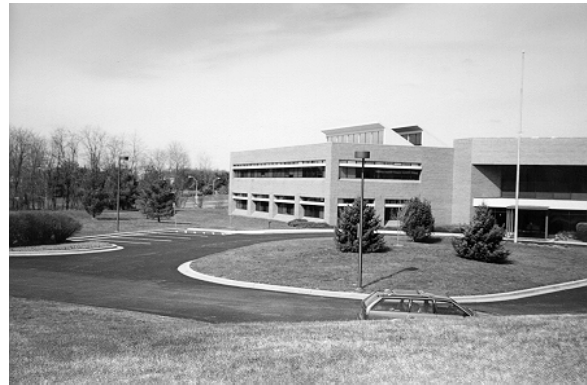
Figure A-24 - View Looking Northwest (Station 4)
