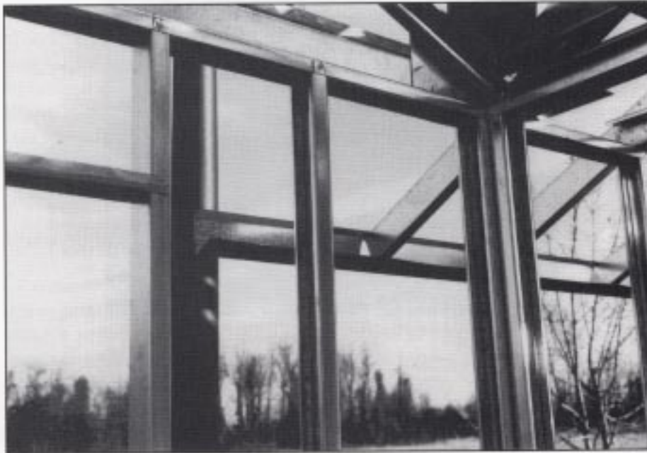
Figure 30 - Stud and track connection
