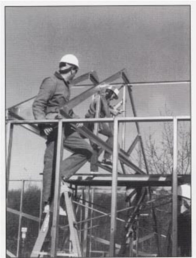
Figure 44 - Setting interior truss
