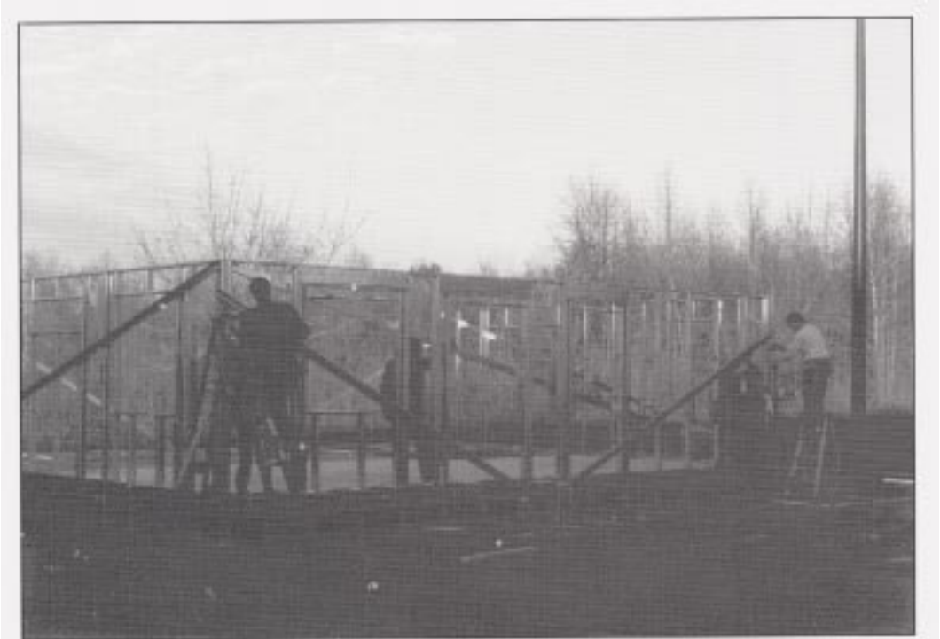
Figure 36 - Panelized wall attachment
