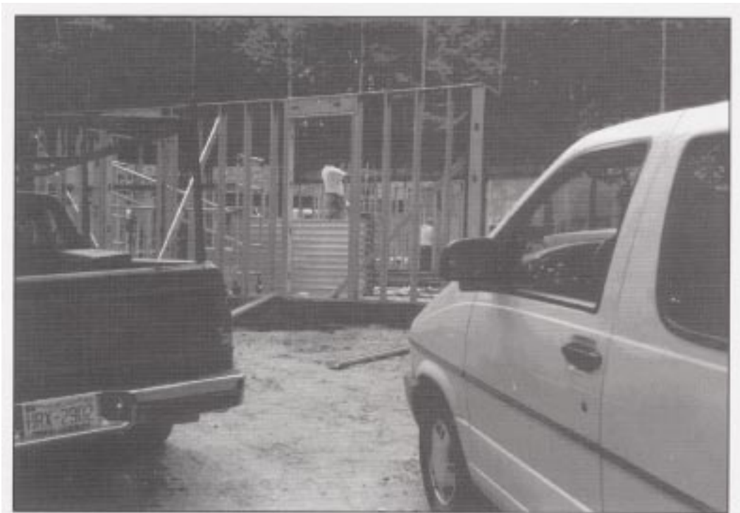
Figure 10 - Installation of basement walls
