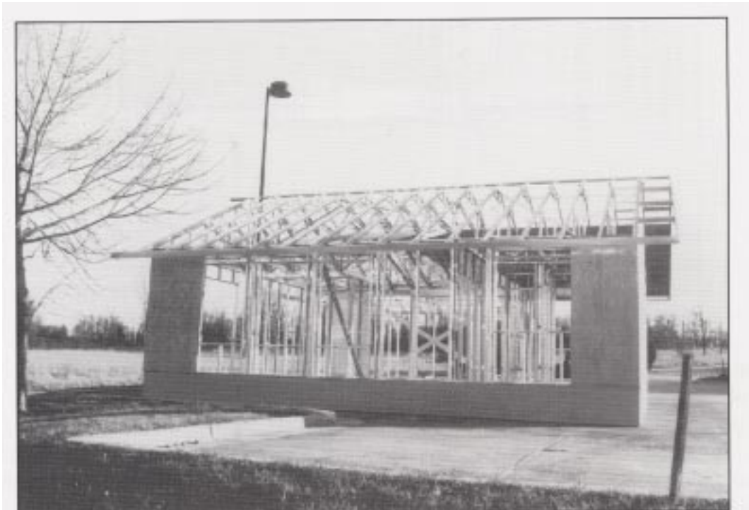
Figure 37 - Plywood wall bracing
