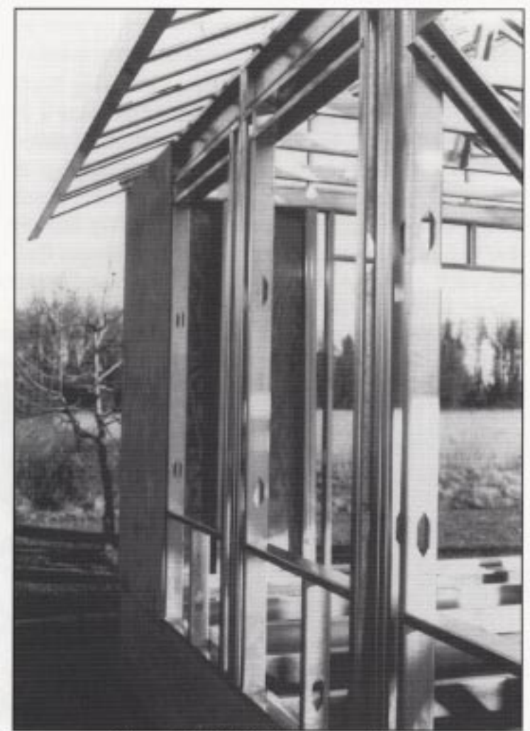
Figure 31 - Wall with aligned holes
