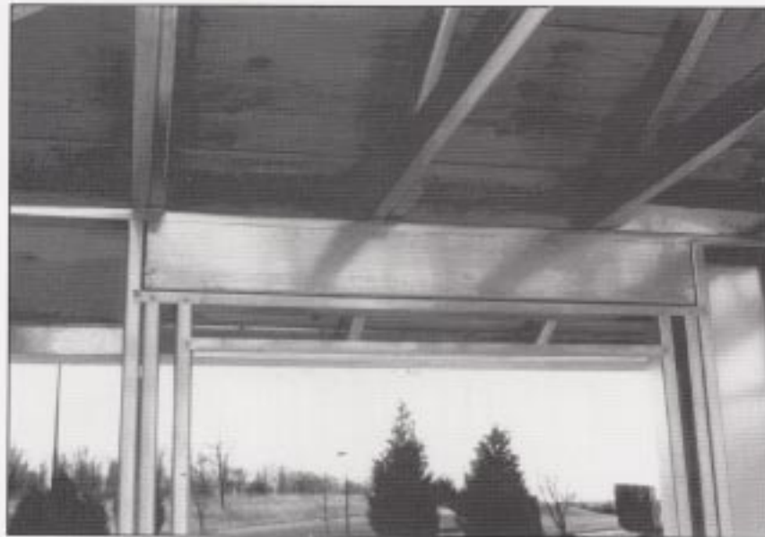
Figure 33 - Box-beam header
