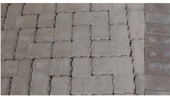
Interlocking permeable pavers
