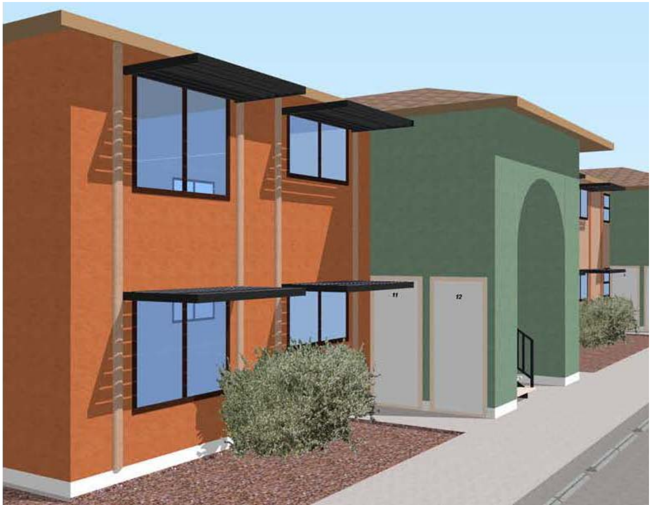
Figure 9: Building B with 4' Louvered Window Shades
