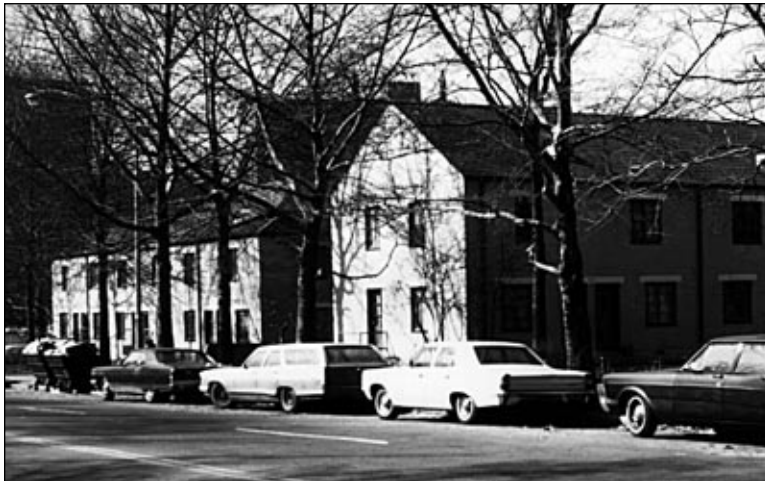
Figure III-1: Clason Point as seen from street, before modifications. Note the overflowing garbage dumpster at left.
