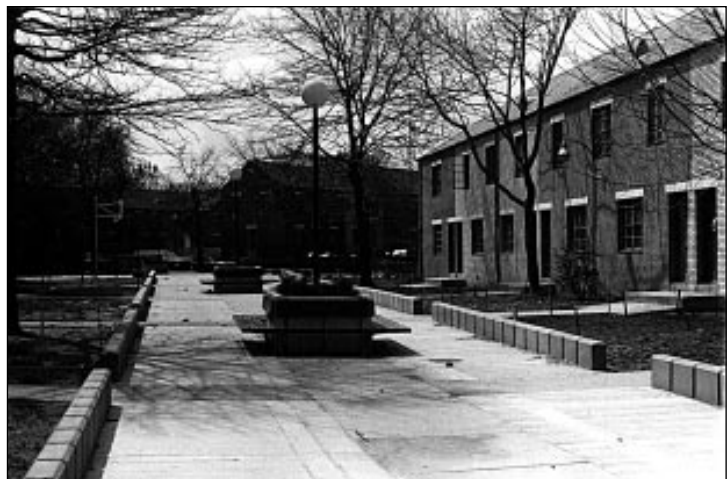
Figure III-5: Collective front yards are defined by the new concrete curbing. A new combination lighting, seating, and planter helps residents use and identify with the central walk.
