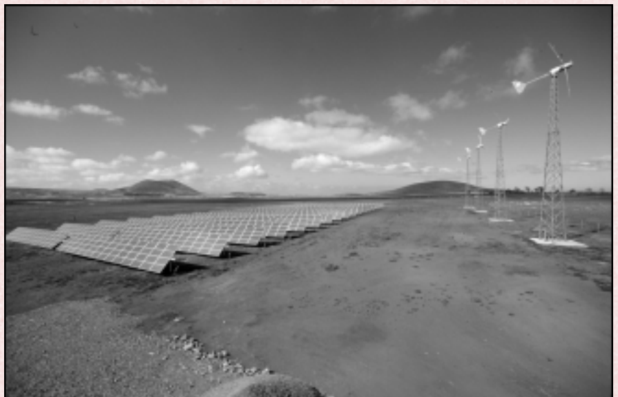
The hybrid solar/wind project at Parker Ranch features 175 kW of solar and 50 kW of wind turbines.
