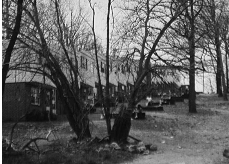
Photo 1.6 Townhouses adjacent to hillside with erosion problem. (David Varady)
