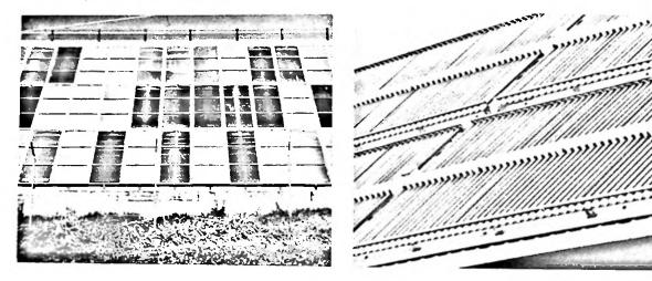
Selective surfaces are not worth the expense when used exclusively with a domestic hot water system. A less expensive coating can provide comparable effectiveness in the range of domestic hot water operating temperatures.
