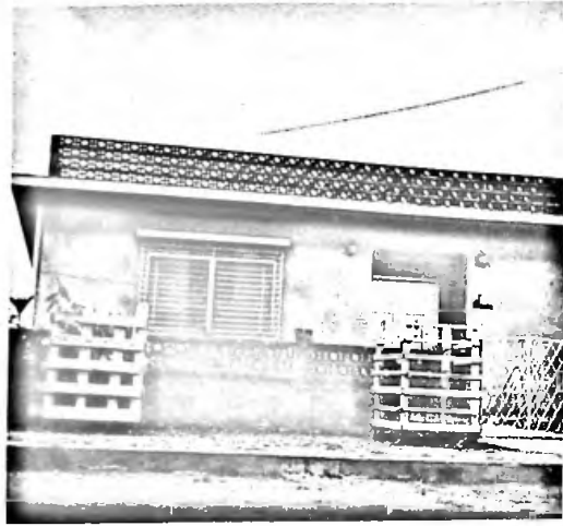
c. Dwelling, near Maracaibo, Venezuela. Open tile parapet permits free ventilation over flat roof while maintaining privacy for personal use.
