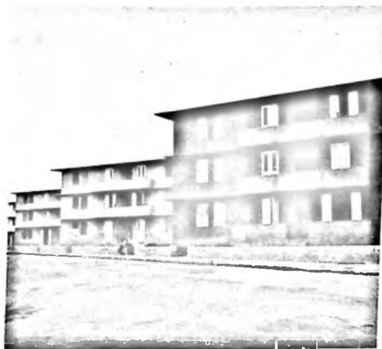
a. Apartment dwellings Puerto Rico. Cross ventilation permitted, but roof ventilation desirable to minimize heating of top story. Advantage not taken of rich natural shade.
