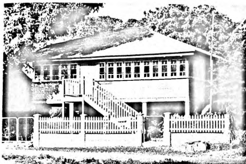
a.—Residence, Townsville, Australia. Verandah almost entirely vitiated by glazing, and internal rooms created. Louvered lower part insufficient compensation. Steps unprotected. (Courtesy, Commonwealth Experimental Building Station.)
