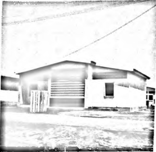
a. New dwelling, Maracaibo, Venezuela. Open tile in wall permits free ventilation while maintaining privacy. Curved tiles permit some ventilation of roof structure. Restoration of natural shade desirable.
