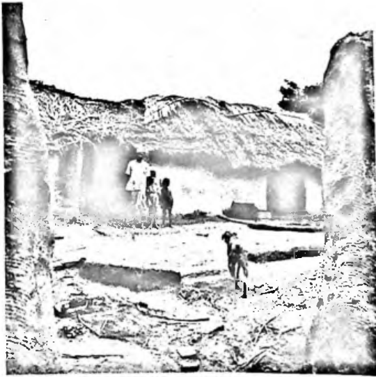
a. "Sweeper's" house, U. P., India. Capacity insulation of mud walls offset by open doorway and dilapidated thatch roof. No through ventilation for warm humid season. Crude drainage for wet season. No opening for escape of smoke. (Photo Lee.)
