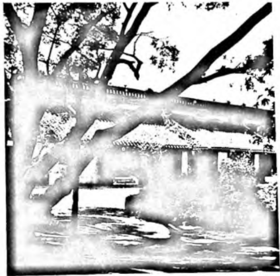
d. Superior residence, Lucknow, India. Wide verandah for wall shade in hot dry, and living space in hot wet season. Heavy construction gives capacity insulation. (Photo Lee.)
