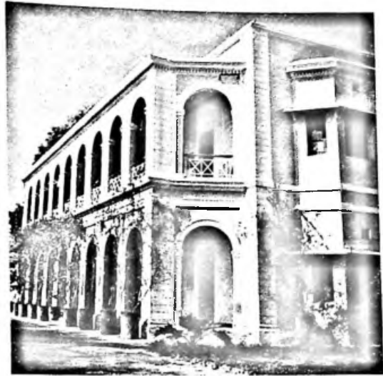
c. Hotel, Lucknow, India. Massive construction gives capacity insulation, but projections insufficient for shade. Ceilings unnecessarily high, making rooms very hard to heat in winter. (Photo Lee.)
