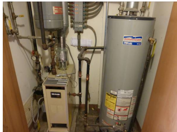
Photo #64: 3 story walk up unit – mechanical equipment
