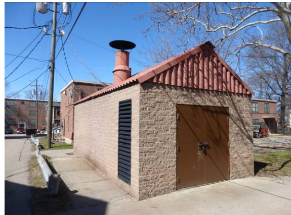
Photo #10: Central boiler house
