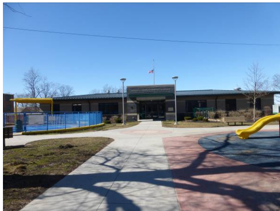
Photo #3: Community center - rear elevation
