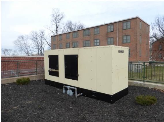
Photo #75: Community center – emergency generator
