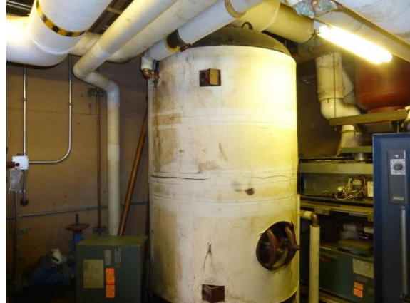
Photo #68: Storage tank
