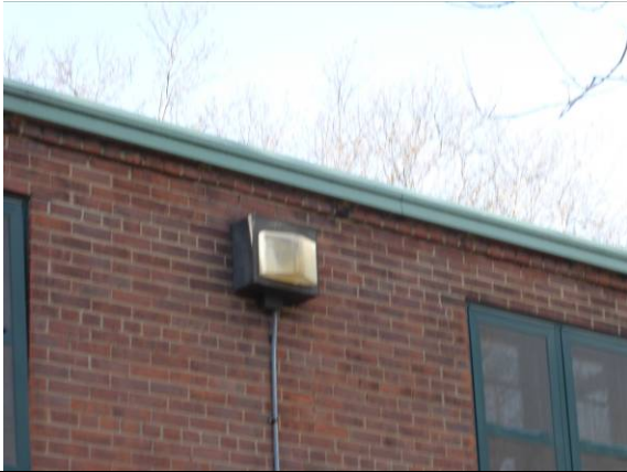
Photo #25: Building mounted site lighting
