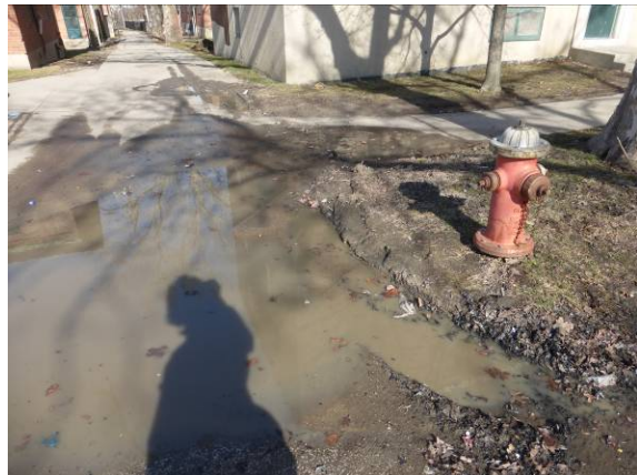
Photo #22: Erosion and ponding issue
