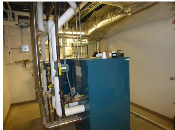
Photo #70: Community Center - boilers
