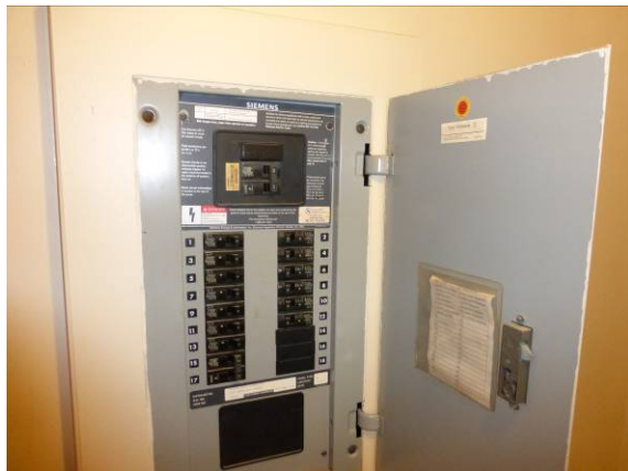
Photo #63: Electrical panel
