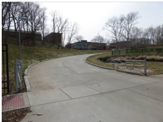
Photo #11: Community center drive way
