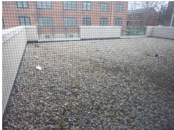
Photo #16: Community center roof
