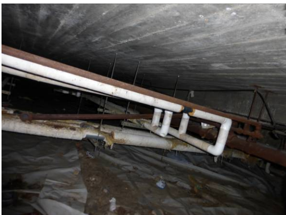
Photo #77: Row-home building crawl space
