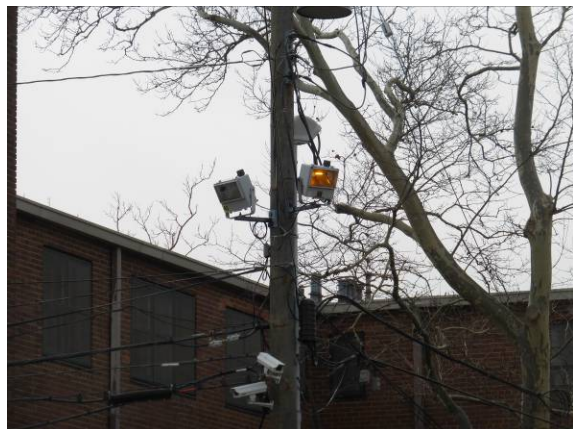
Photo #24: Site lighting
