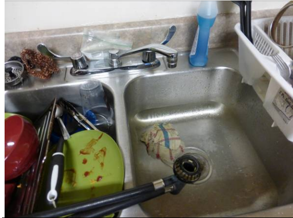
Photo #50: Washer hookup to kitchen sink
