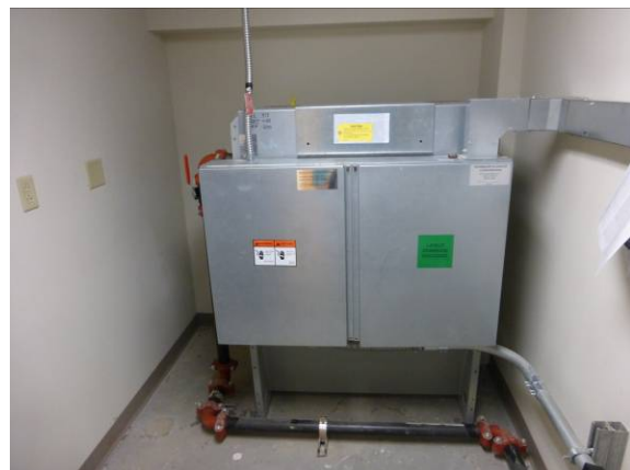
Photo #72: Community center - hydraulic elevator equipment
