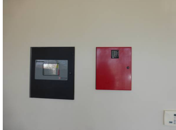
Photo #74: Community center – fire panels
