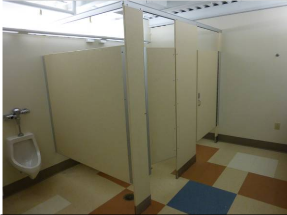
Photo #37: Community center - bathroom
