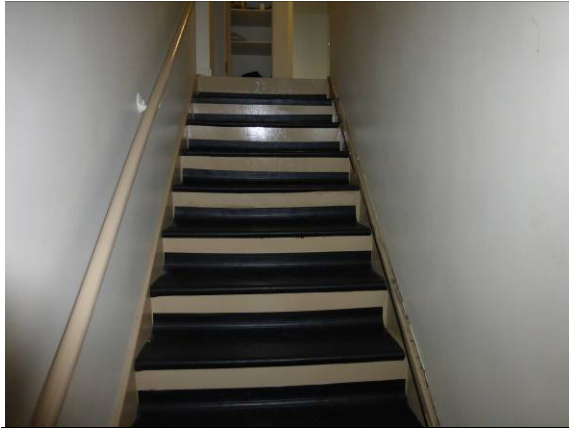
Photo #55: Interior stairs
