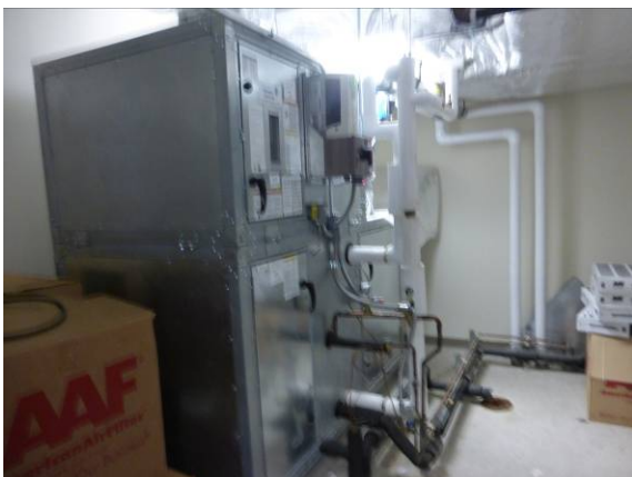
Photo #71: Community center - air handler
