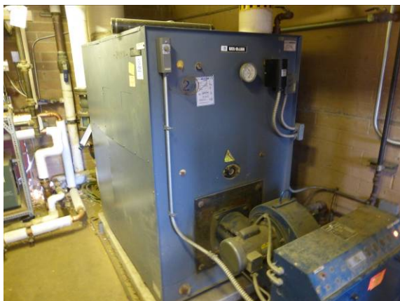
Photo #65: Central heating boiler
