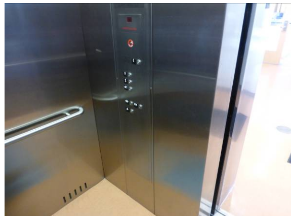
Photo #34: Community center - elevator
