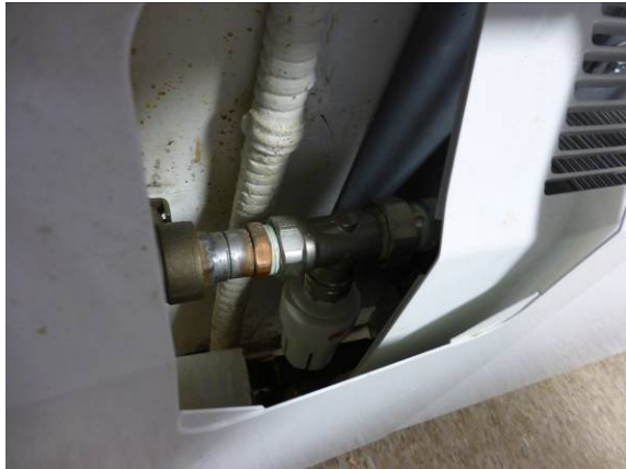
Photo #61: Radiator control
