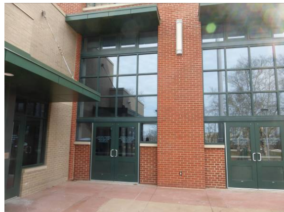
Photo #30: Community center - exterior doors and windows
