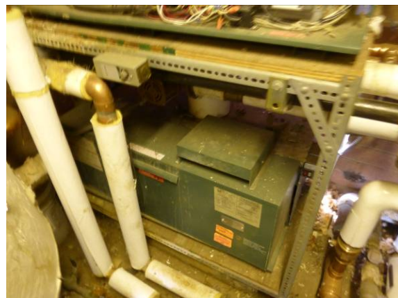
Photo #66: Central domestic water boiler
