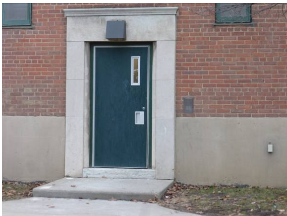
Photo #29: 3 story walk up - exterior door
