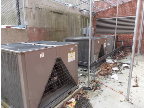
Photo #73: Community center – split system units
