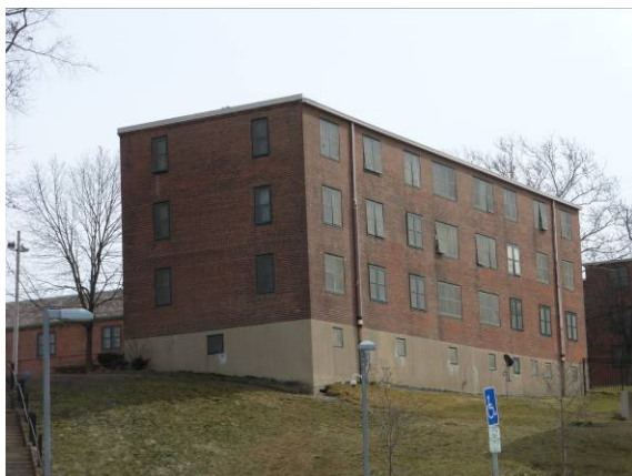
Photo #5: 3 story walk up - rear elevation
