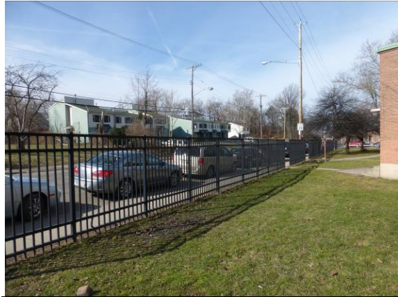
Photo #20: Perimeter fencing
