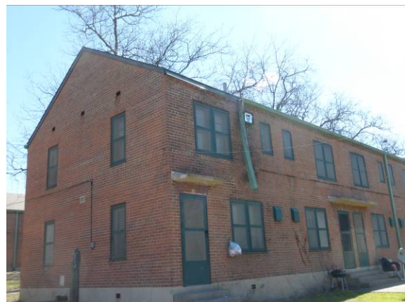
Photo #6: Pitched roof row homes - front and side elevation
