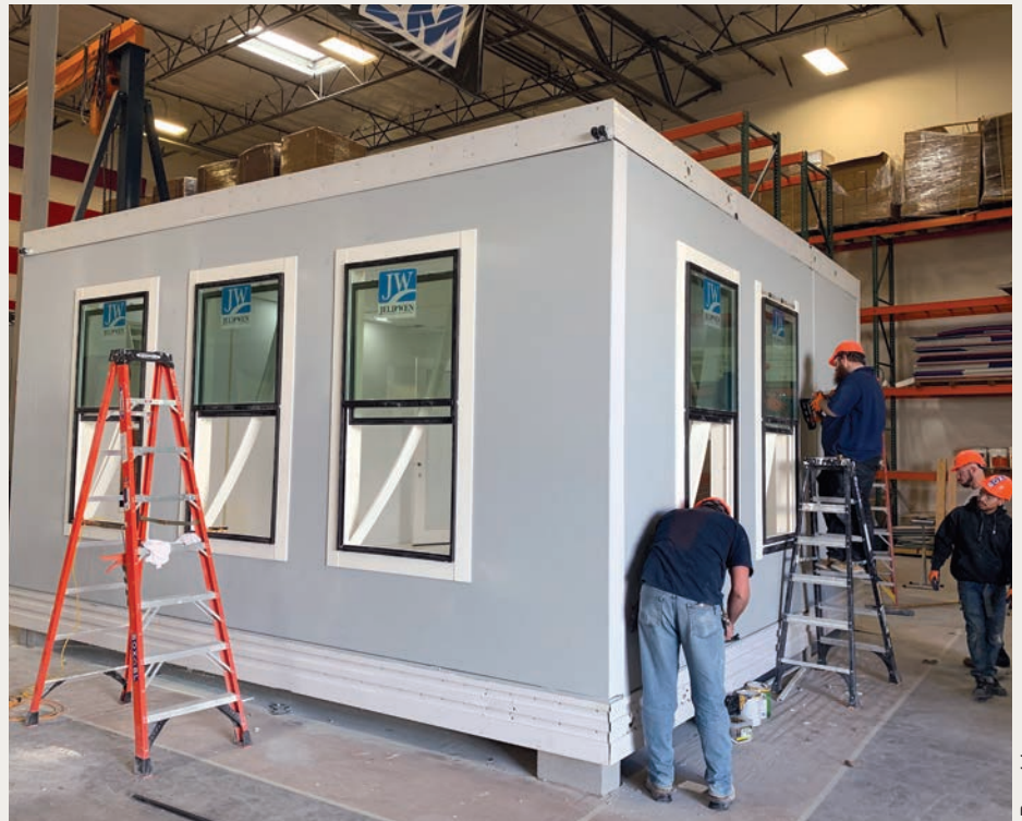
ADU under construction.
