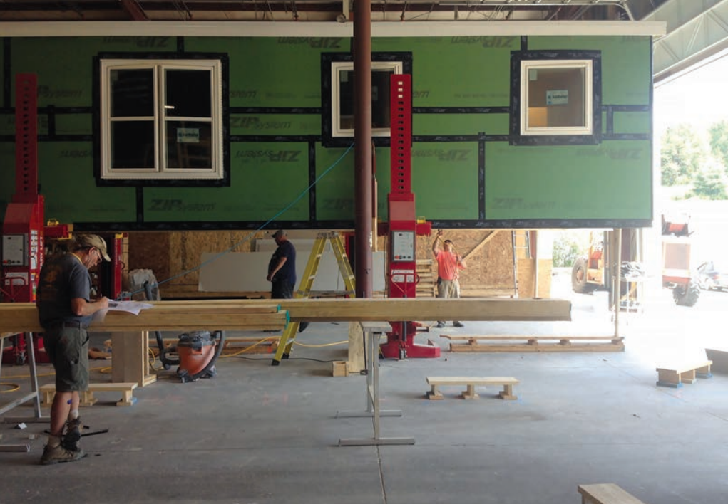
Constructing ZEM homes inside the Vermod factory reduces weather-related delays and provides stable working conditions for employees.
