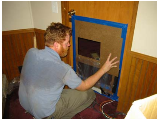
Figure 3-9 Adjusting the return air opening size through a bedroom door
