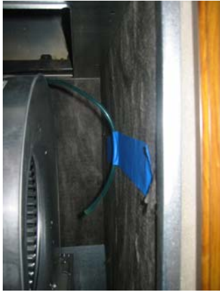
Figure 2-5 Pressure probe at air handler fan
