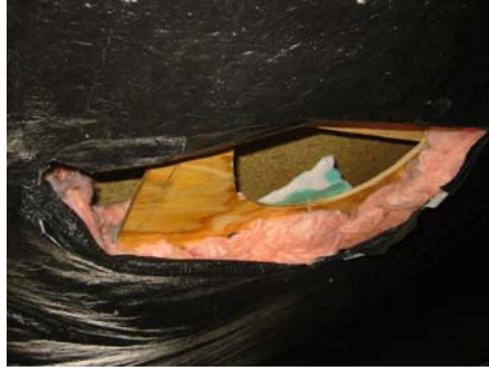
Figure 2-12 Bottom board hole in single section home
