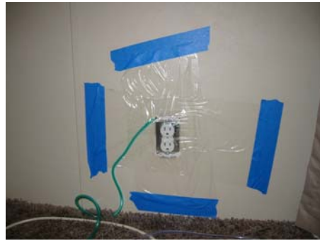
Figure 2-6 Pressure probe in wall
