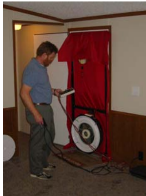
Figure 2-9 Measuring shell leakage with a blower door
