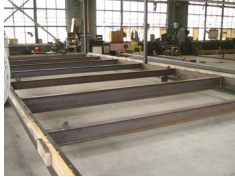
Figure 51 Floor frame for concrete floor module
