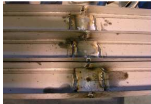
Figure 32 Welded wall track
