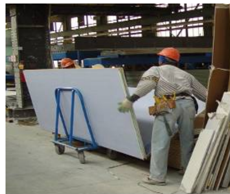
Figure 29 Loading gypsum board on a cart
