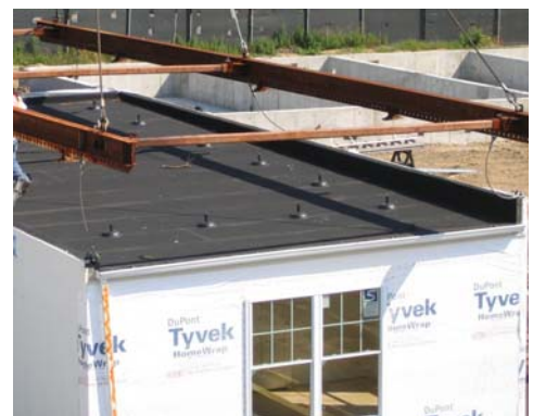
Figure 55 Triangular parapet wall
