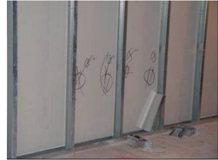
Figure 46 Relocating an electrical box
