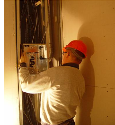
Figure 27 Installing an electrical panel
