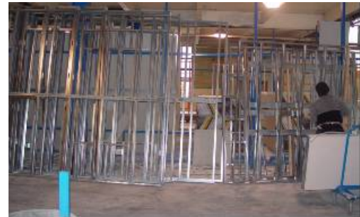
Figure 47 Wall frames ready for gypsum board
