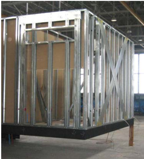
Figure 2-11 Portion of framed home section showing cross-bracing and header
