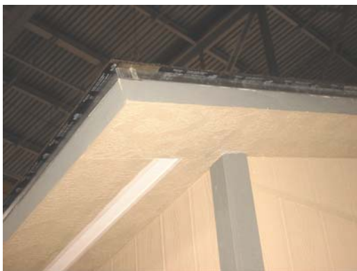
Figure 2-22 The eave overhang with soffit vent
