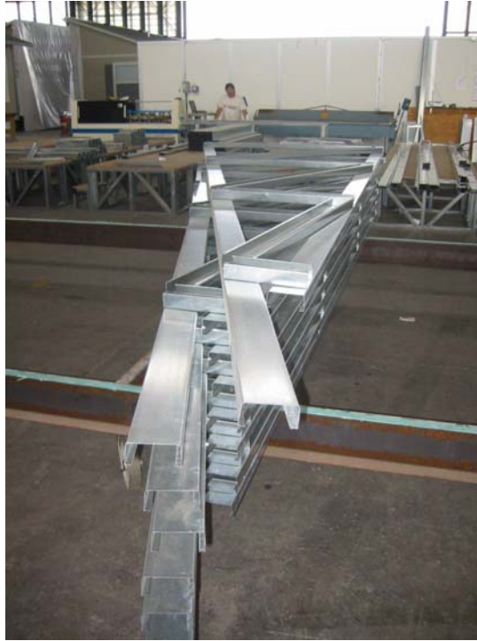
Figure 2-6 Assembled steel roof trusses
