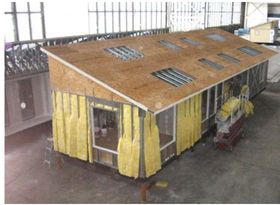
Figure 2-10 Insulation being placed in assembled home section
