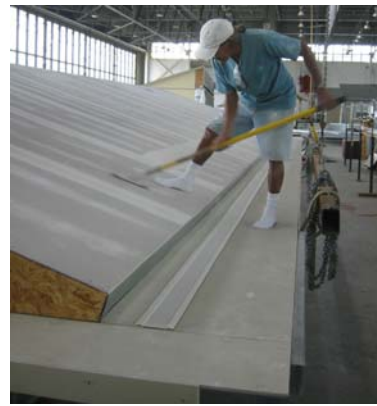
Figure 2-8 Gypsum board applied to the ceiling
