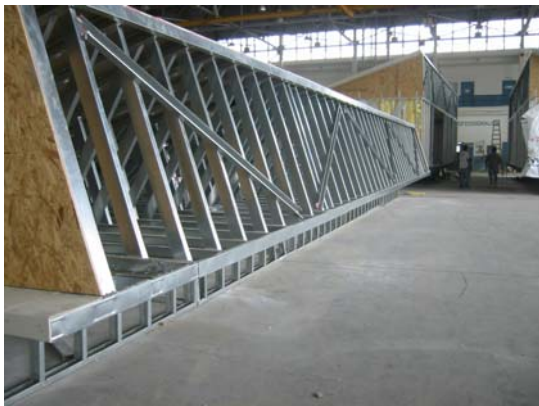
Figure 2-7 Roof assembly
