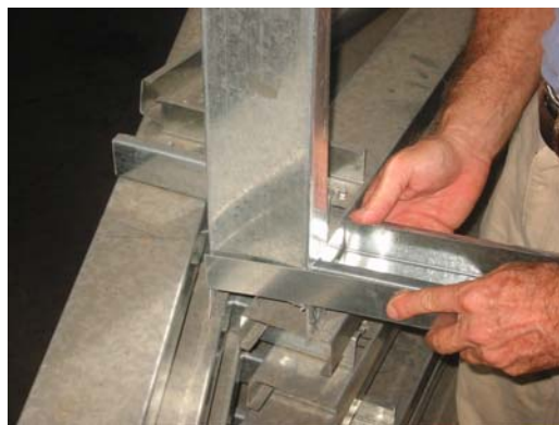
Figure 2-23 Connection of the truss to the wall studs
