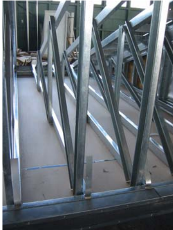
Figure 2-18 Roof trusses being connected to the ceiling board
