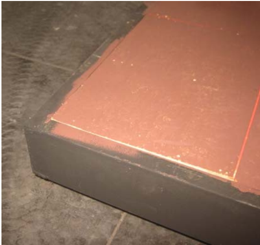
Figure 2-40 Top of floor decking in same plane as top of chassis channel
