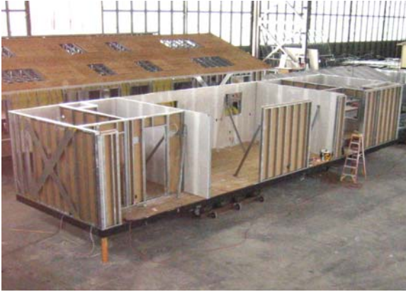
Figure 2-9 Home section prior to roof installation
