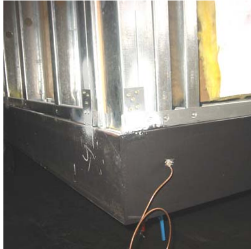
Figure 2-41 Detail of wall framing at chassis edge
