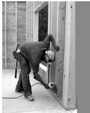
Fig. 3.32: Nailing to adjacent panel
