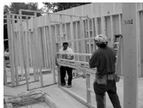
Fig. 3.33: Carrying interior unsheathed wall panel
