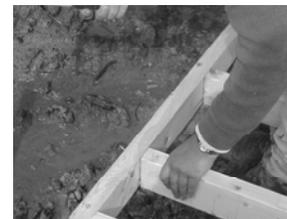
Fig. 3.54: Repositioning stud to avoid interference with anchor bolt
