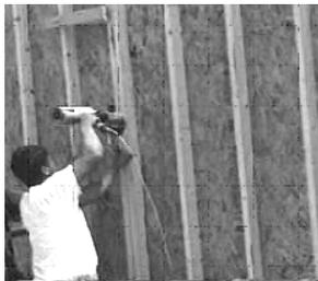
Fig. 3.45: Anchor nailing into position
