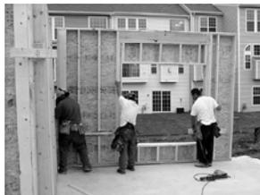
Fig. 3.28: Adjusting panel to slab marks
