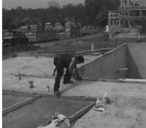
Fig. 3.41: Sill seal gasket installed on slab
