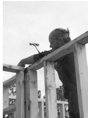
Fig. 3.56: Tying top plates together
