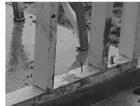
Fig. 3.55: Cut nail temporary anchors
