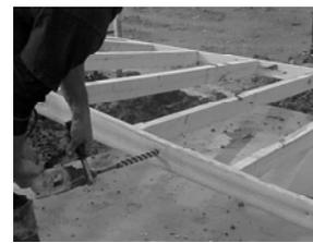
Fig. 3.51: Drilling baseplate for anchor bolt clearance, sill seal gasket in place
