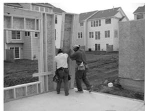
Fig. 3.31: Placing small exterior closure panel
