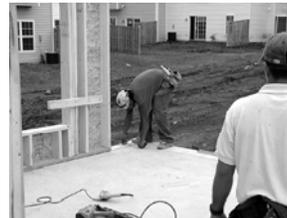
Fig. 3.19: Locating anchor bolt at slab edge
