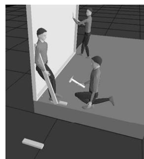
Fig. 2.13: Ergo team plumbs panel, adjusts panel plumb with a back, and nail brace into position at floor cleat
