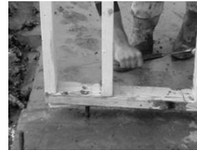
Fig. 3.52: Seating wall panel over anchor bolt
