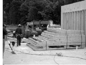
Fig. 3.15: Palletized wall panels as delivered to townhouse slab
