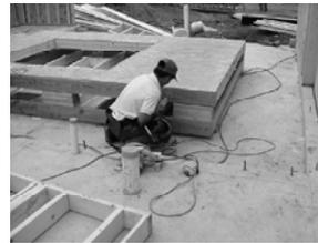
Fig. 3.21: Drilling anchor bolt holes in panel
