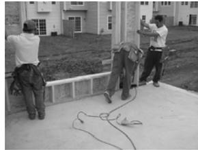
Fig. 3.30: Anchor nailing into position
