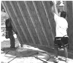
Fig. 3.44: Nailing to adjacent panel
