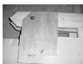
Fig. 3.9: Hinged connection between rafter and joist
