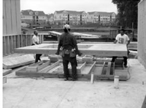
Fig. 3.24: Preparing to lift panel vertical
