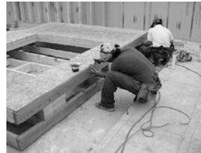
Fig. 3.20: Transferring anchor bolt locations to bottom plate of wall panel
