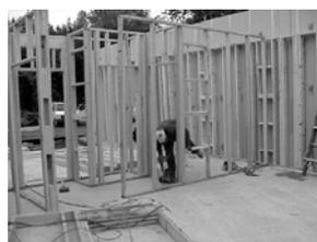
Fig. 3.34: Anchor nailing interior panel to slab
