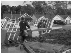
Fig. 3.49: Two workers move a wall panel to the slab
