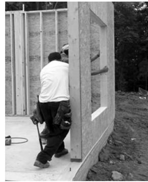
Fig. 3.29: Placing panel over anchor bolts
