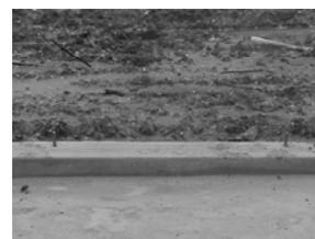
Fig. 3.57: Anchor bolts set too close to slab edge for flush fit between foundation and OSB sheathing
