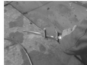
Fig. 3.53: Cutting off misplaced anchor bolt
