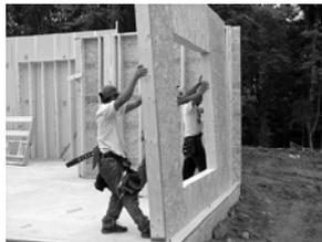
Fig. 3.27: Seating over anchor bolts
