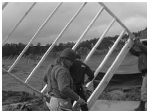
Fig. 3.50: Transferring anchor bolt location to panel
