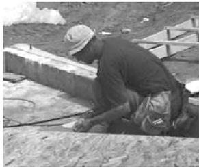
Fig. 3.43: Carrying sheathed panel to slab location
