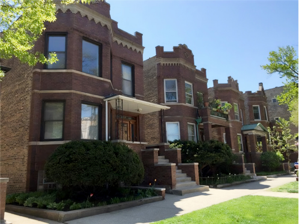
A block with two- to four-unit buildings in Chicago. Photo credit: Institute for Housing Studies at DePaul University.
