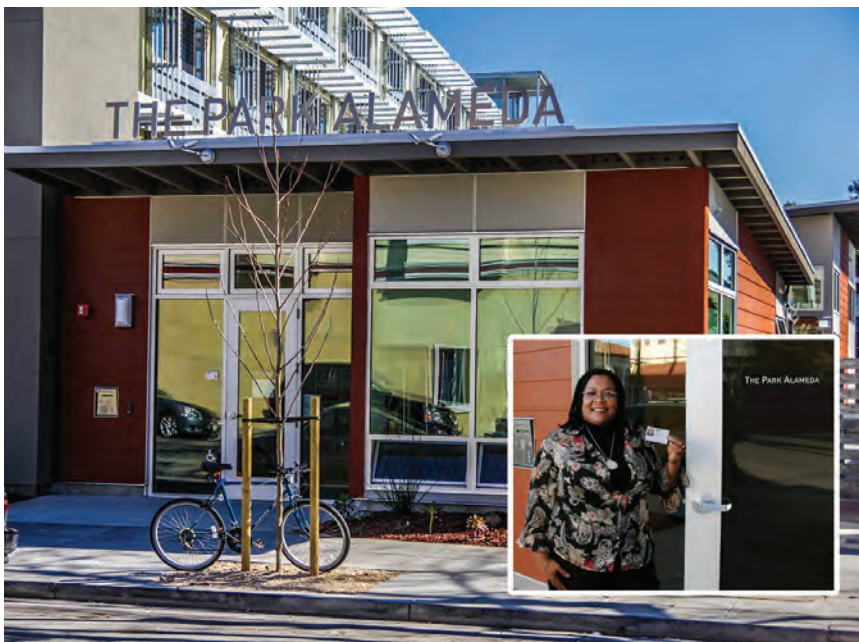
Figure 33. The Park Alameda; resident with a new EasyPass bus pass (inset). The Park Alameda, which was formerly a motel, is a 62-unit affordable housing development in the small city of Alameda, California. The project is located in Alameda's historic downtown district, which offers excellent bus service and jobs, retail, and services located within walking distance. The developer, Resources for Community Development, joined the local transit agency's EasyPass program, which provides discounted bus passes for all residents. The project also includes green and sustainable features such as insulated low-emissivity windows and water-heating solar thermal collectors.
