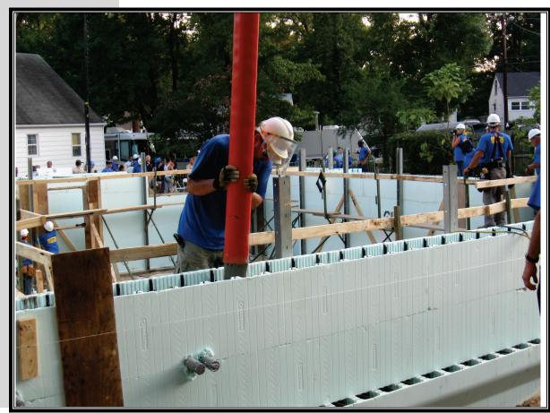
FIGURE 1.5 House Construction Using Insulating Concrete Forms
