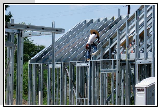
FIGURE 1.4 House Construction Using Cold-Formed Steel Framing
