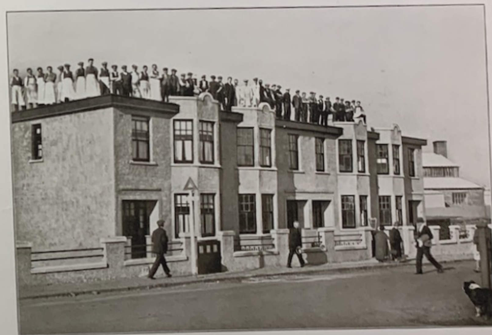
A TESTIMONY TO THE STABILITY OF THIS FLAT-ROOFED CONSTRUCTION—OVER FORTY WORKMEN ON THE ROOF OF THIS BLOCK OF HOUSES.
