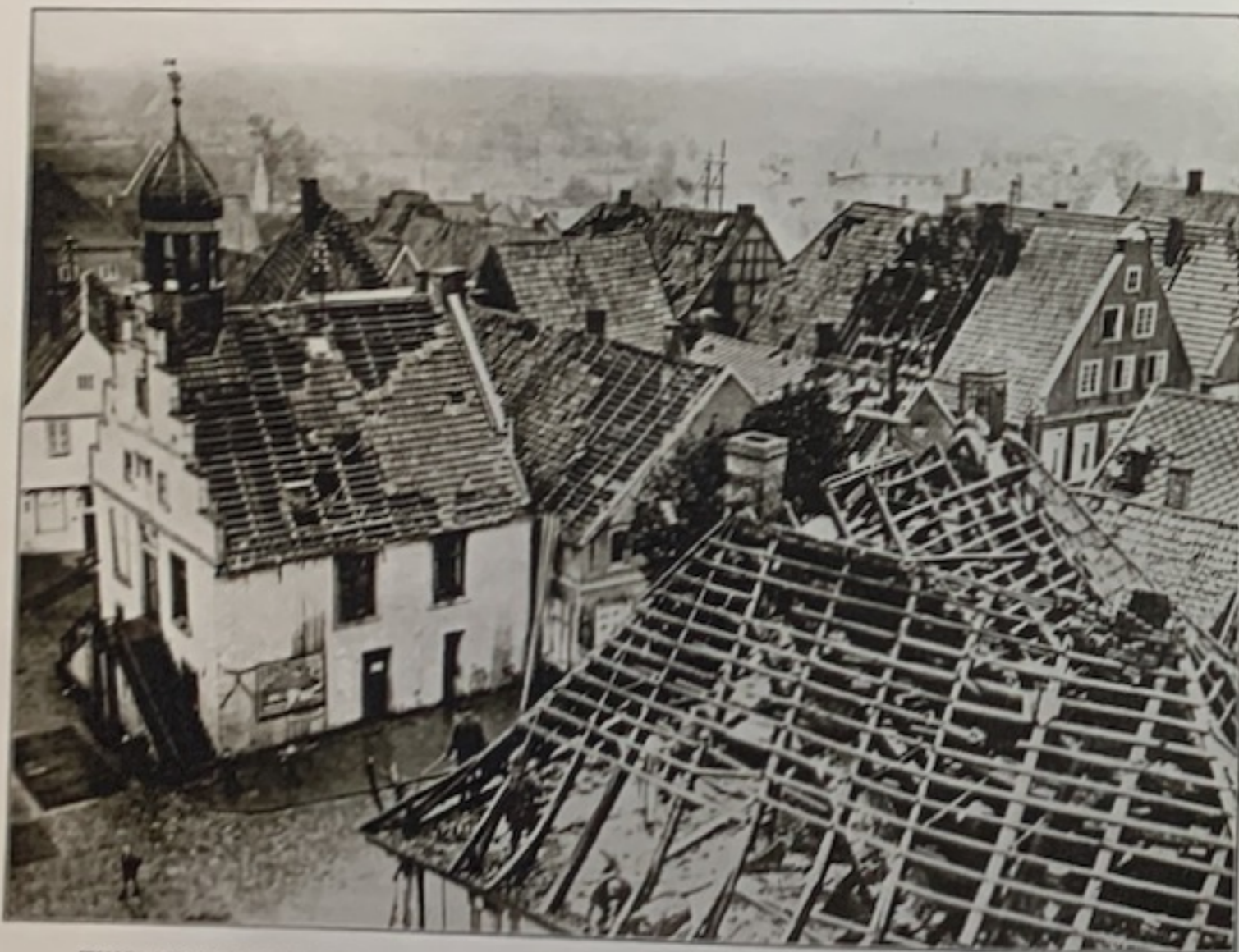
THIS PHOTOGRAPH SHOWS TILED ROOFS COMPLETELY STRIPPED BY A STORM OF VERY MODERATE STRENGTH; IF THERE HAD BEEN ANY GREAT FORCE OF WIND, SOME ROOF-TIMBERS OR WALLS WOULD HAVE FALLEN, BUT THESE ARE ALL INTACT, THE TILES HAVING BEEN SIMPLY STRIPPED OFF.
