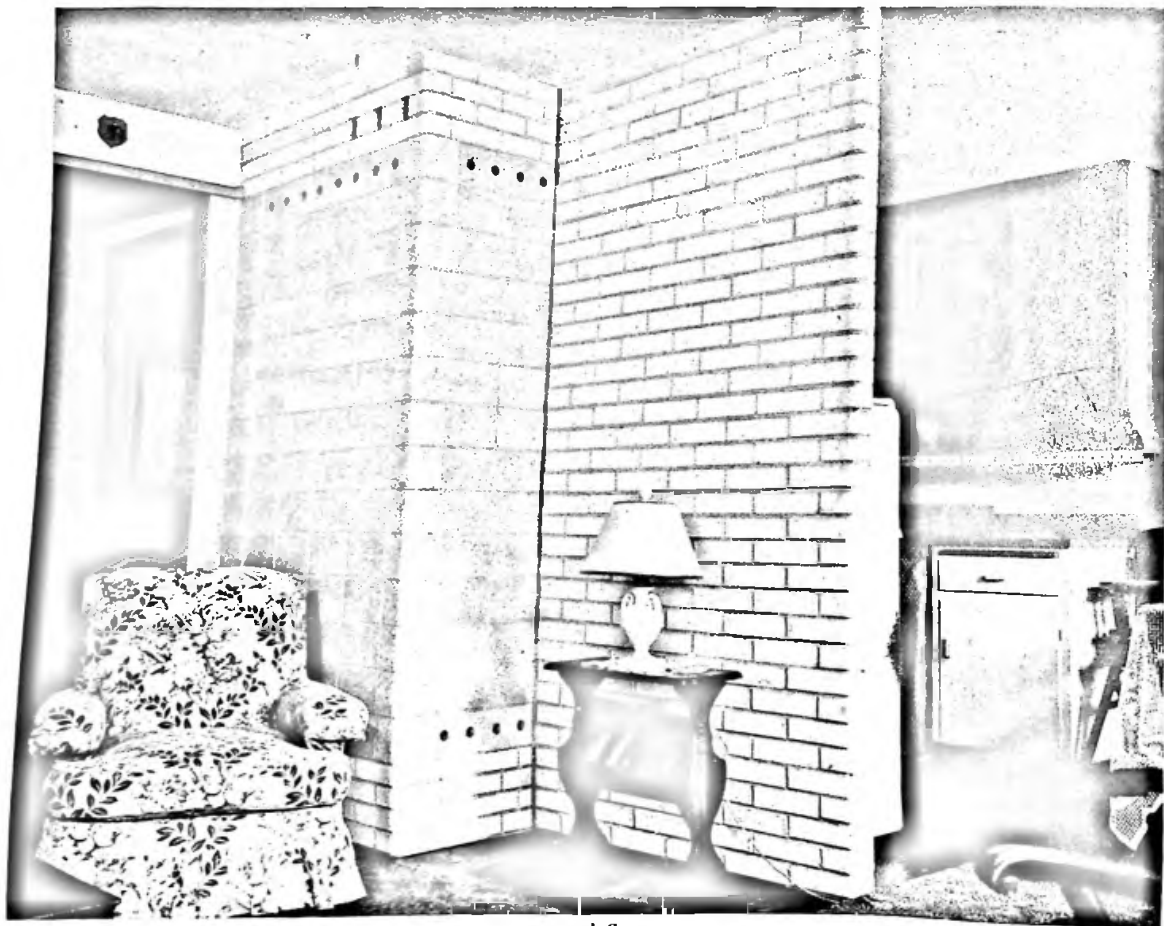
Flue from ceramic heater also warms rooms on second floor
