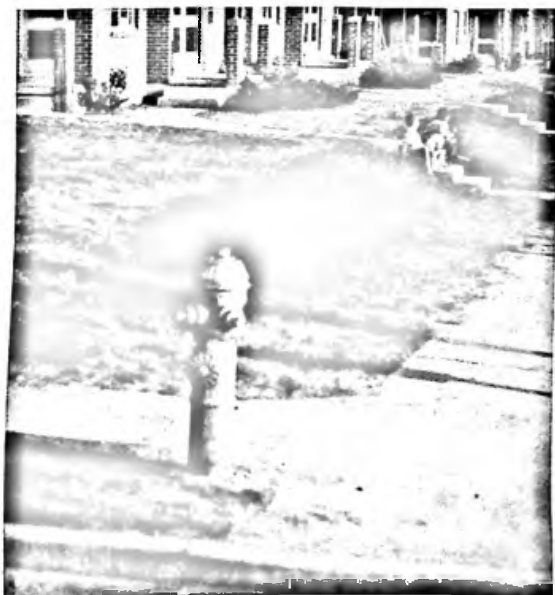
Hydrants should be set to finished grade
