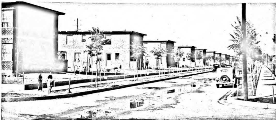
The dished section is undesirable for streets and main drives
