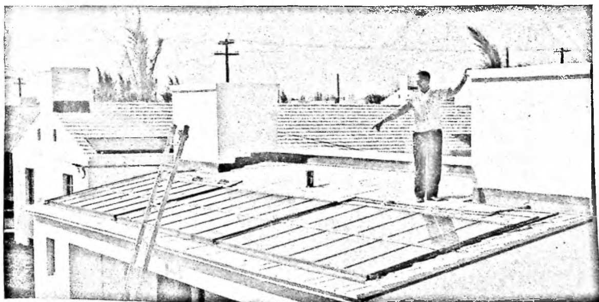
The direct method is used where there is no danger of freezing
