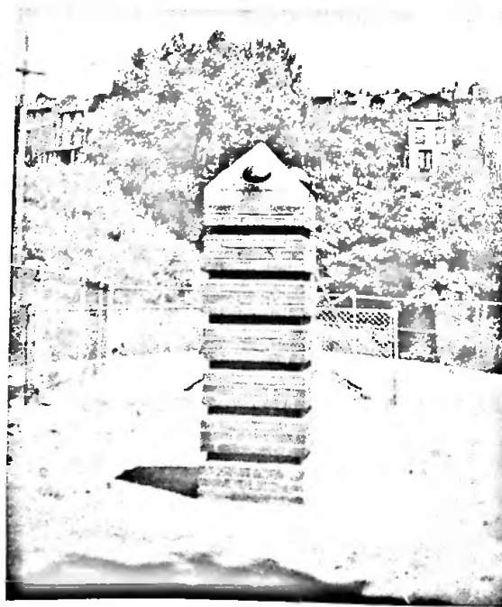
Substantial spray head standard affording unobstructed spray
