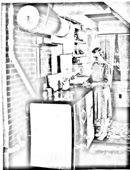
Cooking, space heating and hot-water heating are here combined
