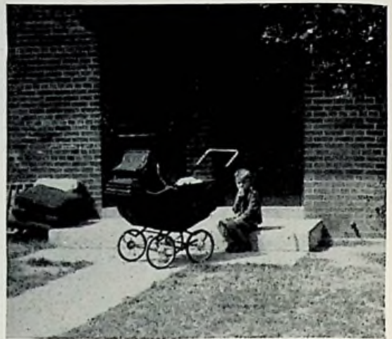
Skimpy pavement results in destruction of bordering grass and in high maintenance costs
