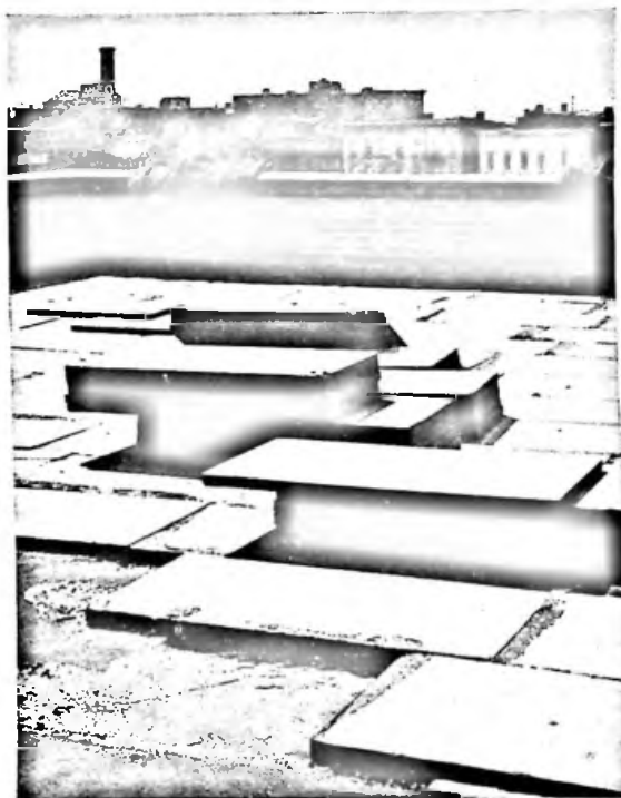
Butted insulation board used on concrete deck
