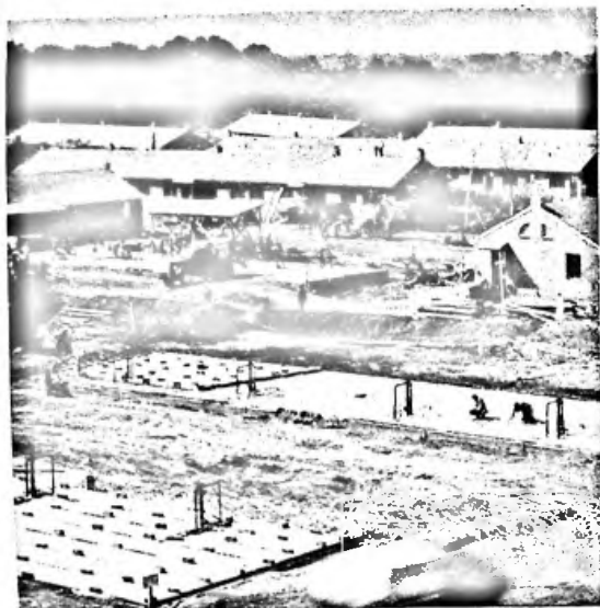
Ground-supported concrete slab is laid over a prepared subgrade
