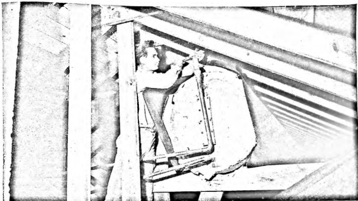
Storage tank hung under the roof
