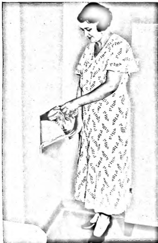
Incinerators off apartment hallways are convenient
