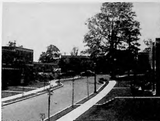
Inaccurate preliminary data resulted in awkward shift in road alignment to save existing tree
