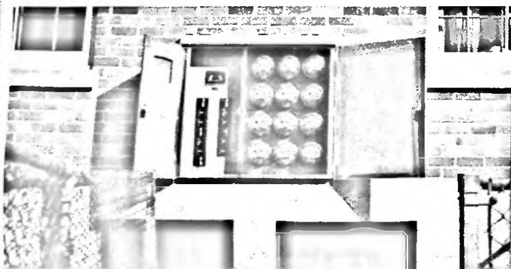
A weatherproof meter cabinet
