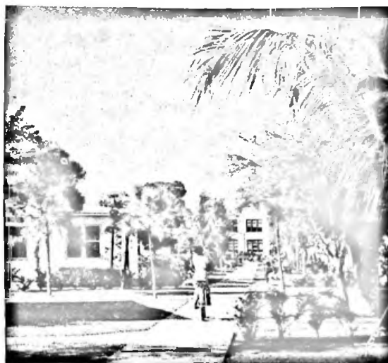
Wavy profile contrasts unfavorably with walkway laid to uniform slope
