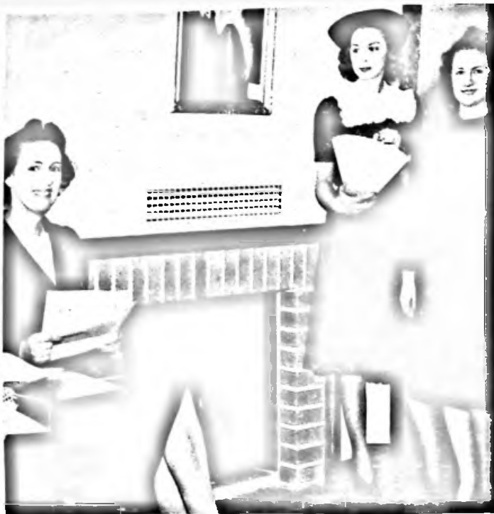
A fireplace with heating grilles may be used in mild climates
