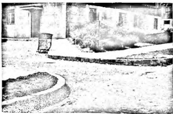
Service drives, cutting sidewalk grade (left) and crossing walk at grade (right)
