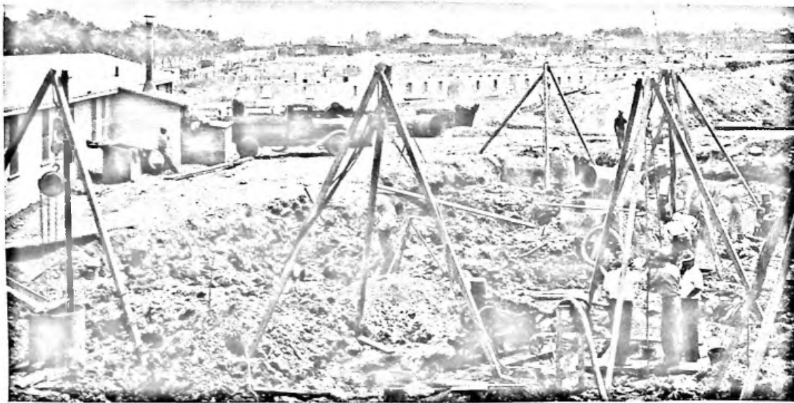
Caissons used in water-bearing soil
