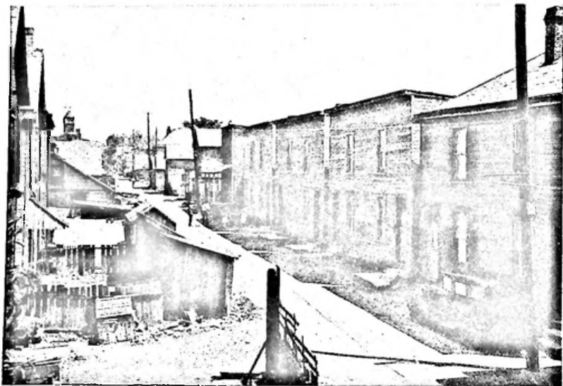
Splintering wooden buildings in Charleston, S. C., and Columbus, Ohio. New low-rent housing, soundly built and permanently protected from blight, will arise in both areas on the sites shown in these photographs.
