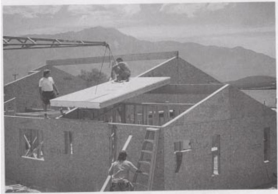
**Photo 6. FOAM-CORE ROOF PANELS BEING SET IN POSITION**
