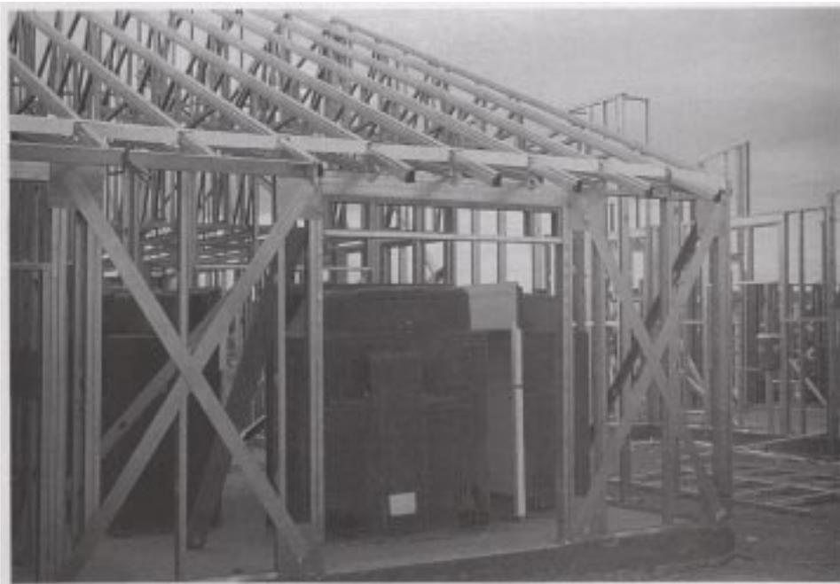
Photo 11. "IN-LINE" FRAMING TECHNIQUE
