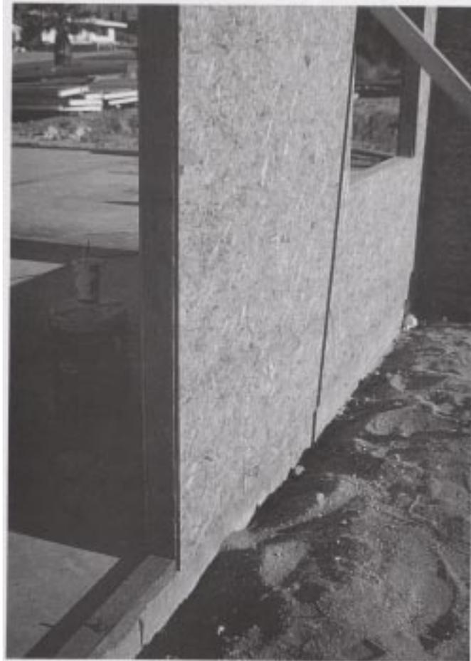
**Photo 3. FOAM-CORE PANEL FASTENED TO SILL PLATE**
