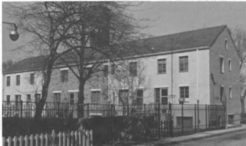
Bronx, N.Y. row houses have served public housing tenants since 1941.
