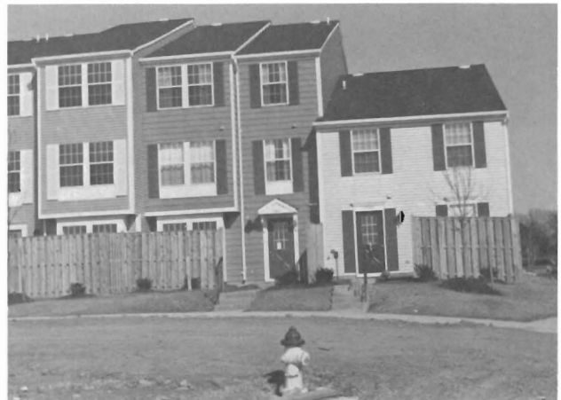
Public housing (middle unit) built as part of a private development in Montgomery Co., Md. in exchange for zoning concessions.
