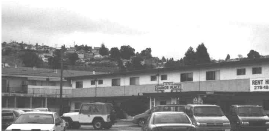
Photo 13. An example of a California motel or doughnut-style apartment development in Ashland, with parking spaces in the center courtyard. (Photograph by David Varady.)
