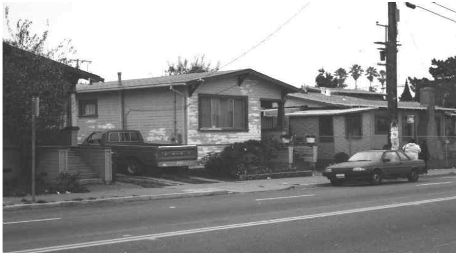
Photo 6. Deteriorated housing in a flatlands neighborhood in Berkeley. (Photograph by David Varady.)
