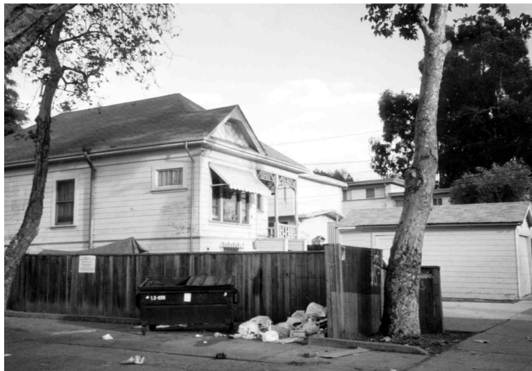
Photo 4. A neighborhood and housing in the Fruitvale section of Oakland showing signs of neglect. (Photograph by David Varady.)
