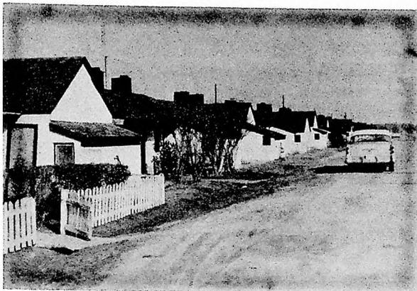
Views looking eastward on Shelter Street show how streets are above floor grade level and how open ditches are provided for drainage.
