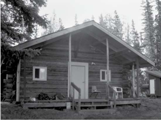
Newly weatherized cabin.
