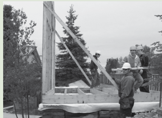
Utilizing construction trades training.
