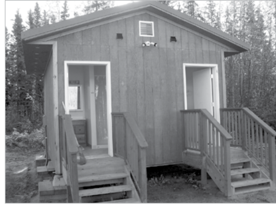
New shower house.
