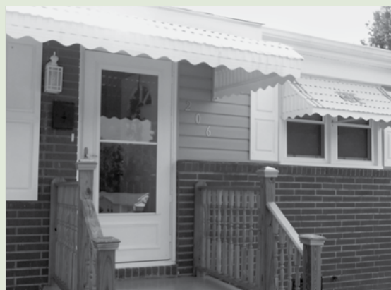
Johnson C. Smith University home rehabilitation project.
