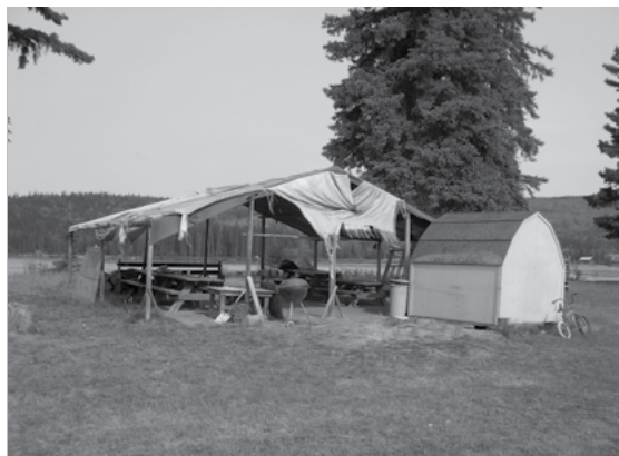
Gaalee'ya Spirit Camp meeting area before renovation.
