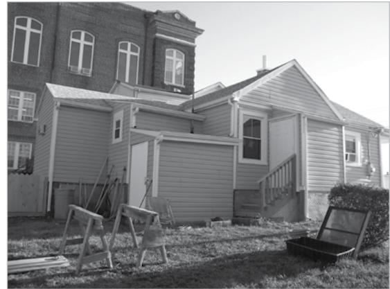
House after rehabilitation project.
