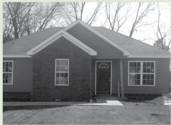
Edmonton Heights home under construction.
