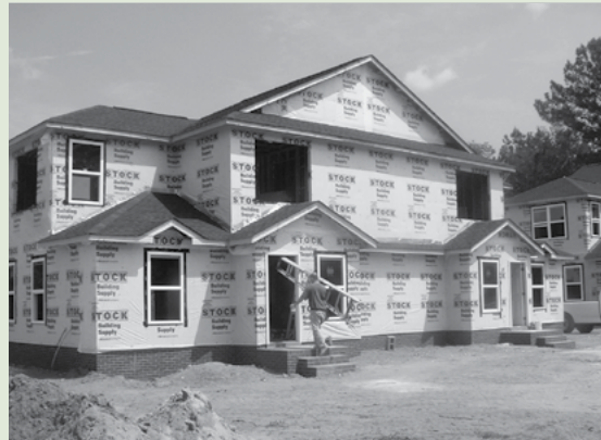
New home construction—unfinished frame.
