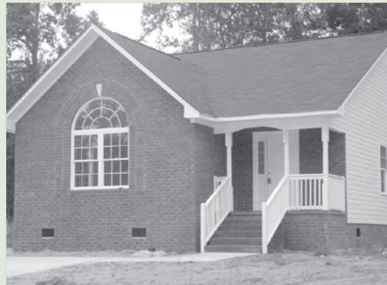
New home constructed under 2006 HUD HBCU grant project.
