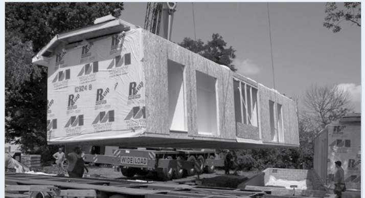
Gracie Jones' modular house is delivered by crane.
