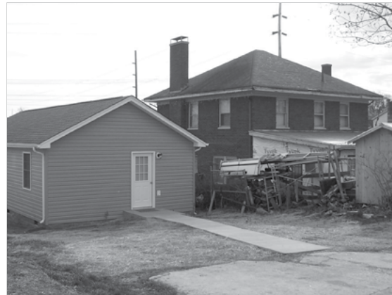
After: Rear view of Cheagle's handicapped-accessible house.
