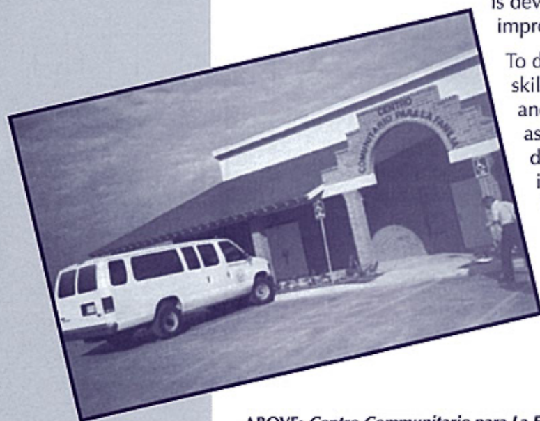
ABOVE: Centro Comunitario para La Familia was constructed with matching funds. COPC funds paid for a transportation analysis and plan.
