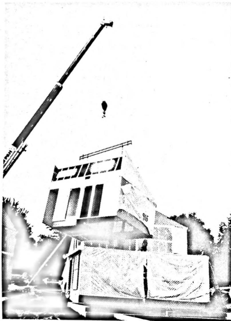
Crane lowering modules
