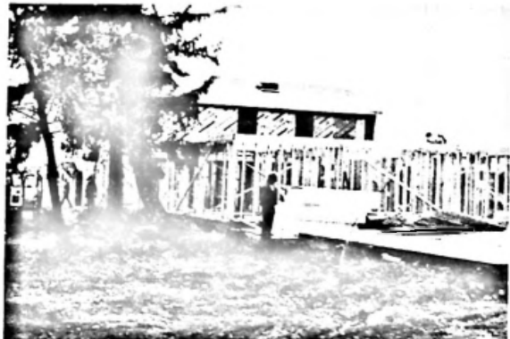
Homes under construction
