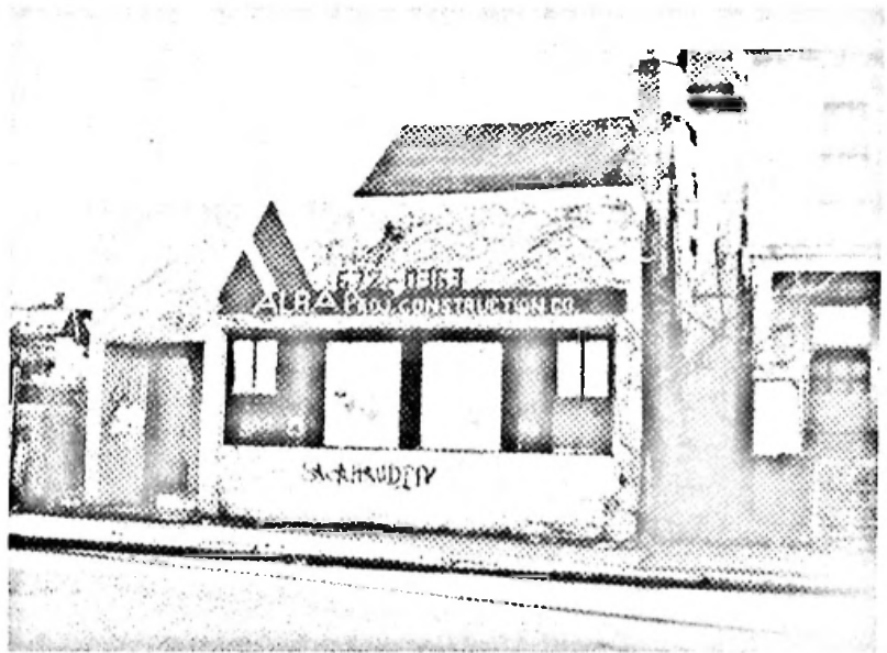
Masonry building removed
