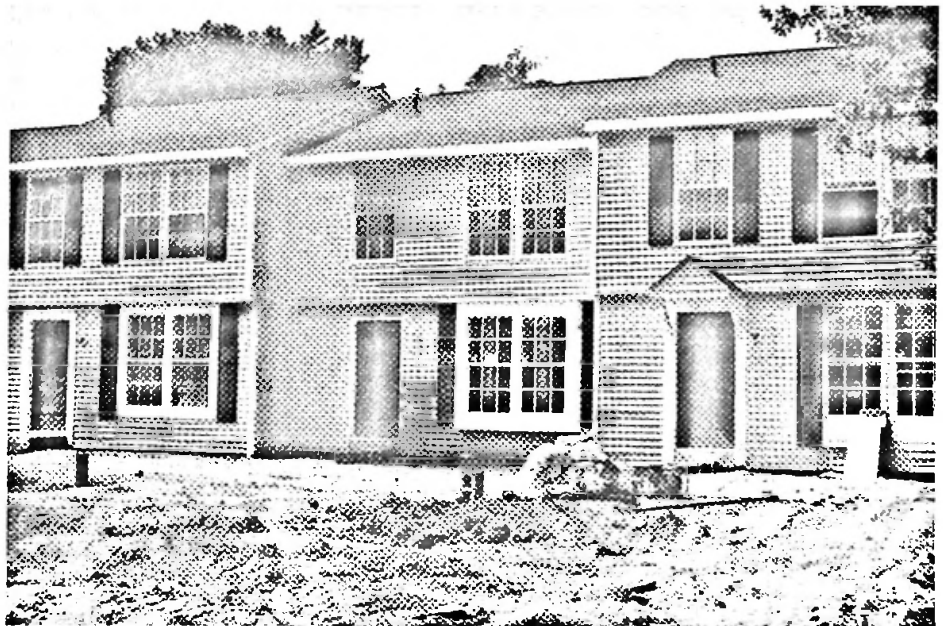
Exterior of modular units
