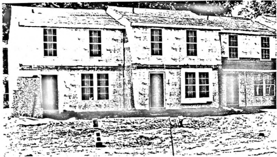
Units delivered without vinyl siding
