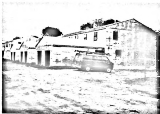
Units under construction
