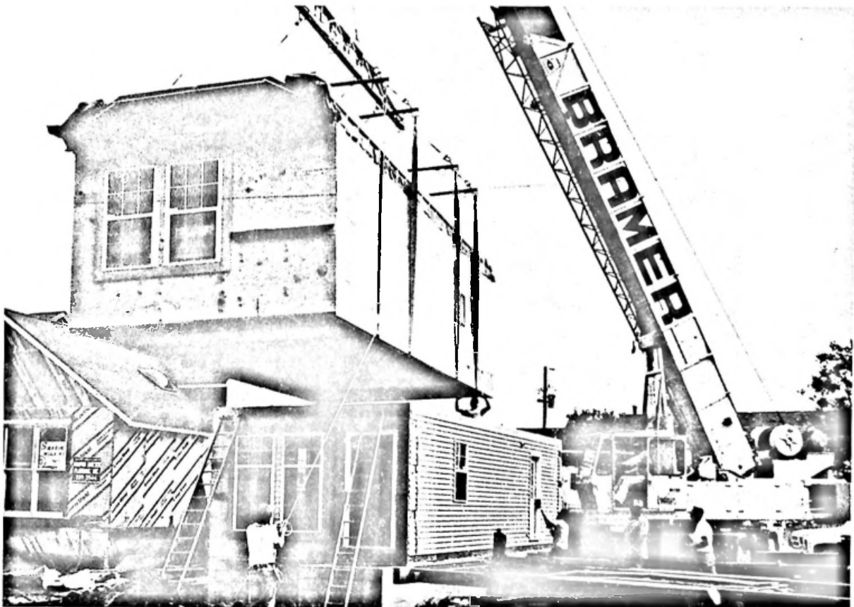
Modular unit being lowered into place
