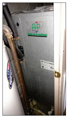
Figure 15: Geothermal Heat Pump, Chester Site Visit
