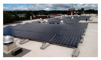
Figure 19: Rooftop Solar Photovoltaic Array, Watervliet Site Visit
