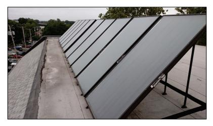
Figure 16: Solar Panels Used for Domestic Hot Water, Chester Site Visit
