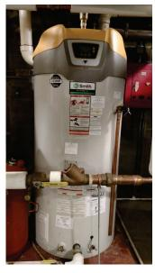
Figure 11: Energy-Efficient Natural Gas Boiler, Wilmington Site Visit
