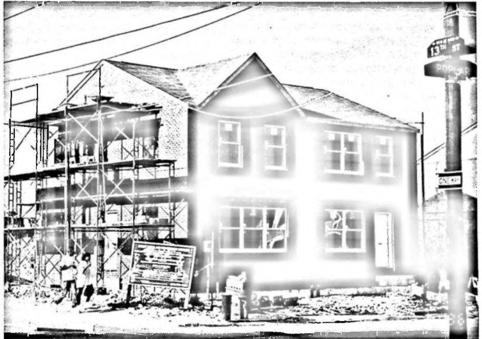
New homeowners under construction: Philadelphia's West Poplar Nehemiah Homes. Some of these homes are now owned by former public housing families.
