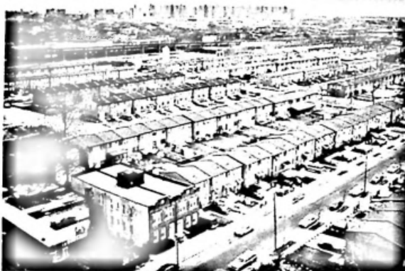
The same Brooklyn neighborhood with Nehemiah townhomes built for affordable homeownership. A majority of the new homeowners are former public housing families.
