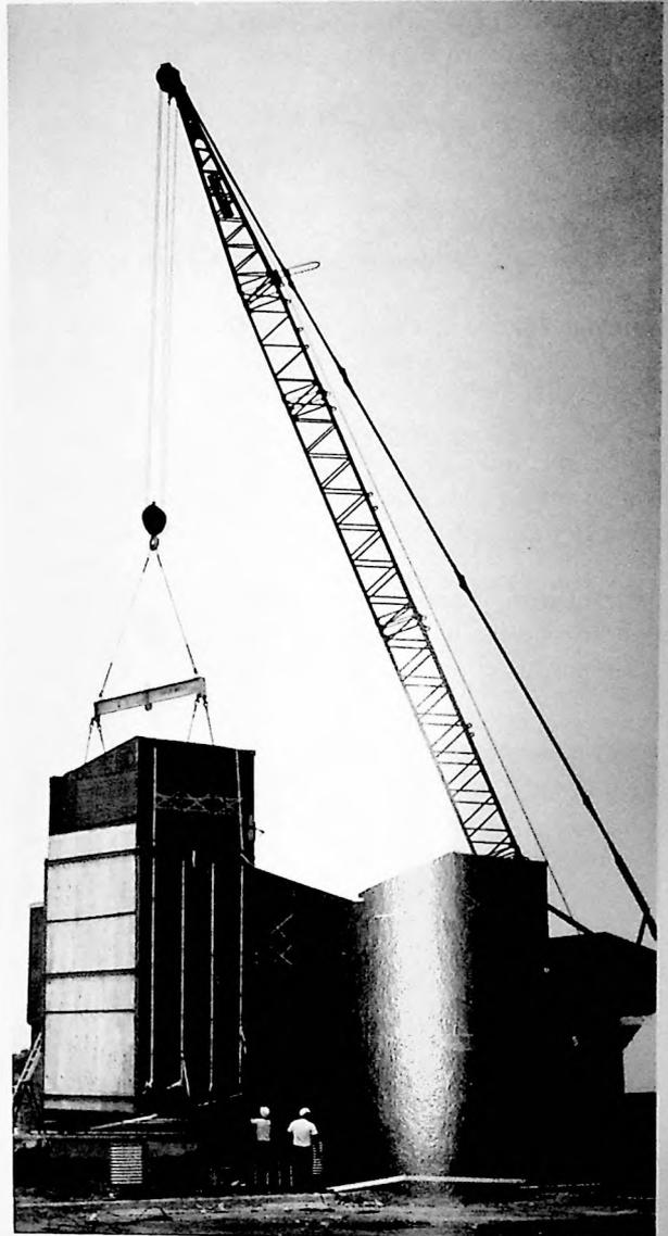
LOWERING "TILT UP" MODULE ON FOUNDATION—HERCULES
