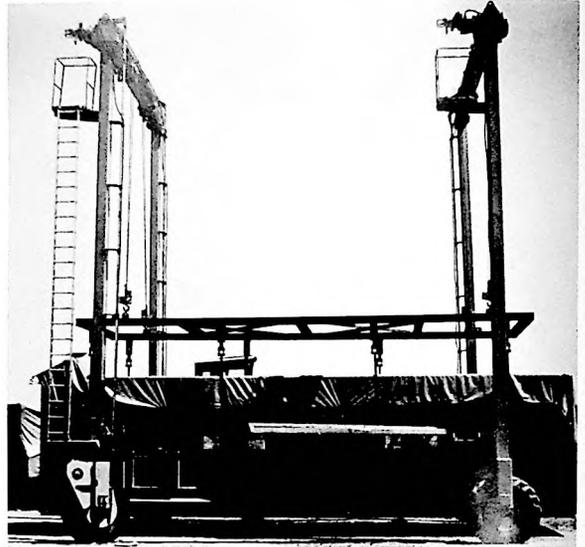
HIGH-LIFT CARRIER POSITIONS HERCOFORM MODULE
