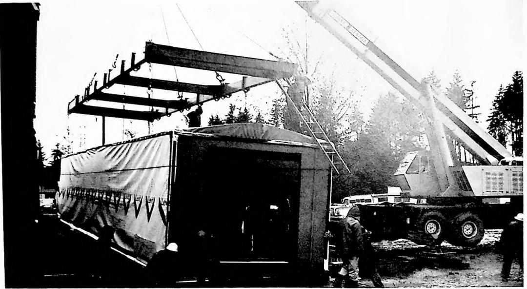
HYDRAULIC CRANE PLACES LEVITT'S FIRST FLOOR MODULE. THESE SIXTY FOOT LONG MODULES WERE INSTALLED WITHOUT DISTURBING THE NATURAL LANDSCAPE.
