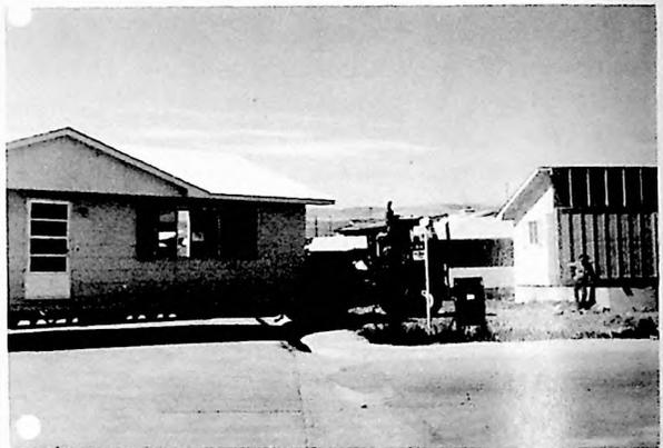
HBC MODULE BEING MOVED ONTO SITE PRIOR TO HORIZONTAL TRANSFER TO FOUNDATION
