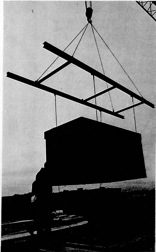
TYPICAL RECTANGULAR SYSTEM WHICH REPLACED THE "DOUBLE-TRIANGLE" SYSTEM
