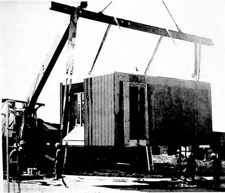
TRUCK MOUNTED 35 TON HYDRAULIC CRANE USED BY GENERAL ELECTRIC TO EMPLACE MODULAR UNITS.
