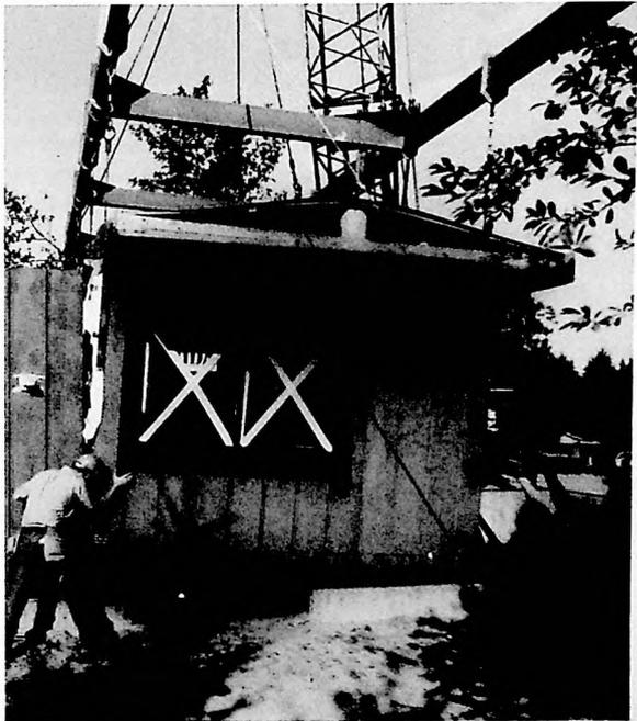
LEVITT FIRST-FLOOR MODULE BEING ERECTED — NOTE TEMPORARY ARCH-SHAPED ROOF
