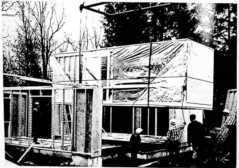
LIFTING AND PLACEMENT OF ALCOA'S MECHANICAL CORE AND ALUMINUM FRAMED WALL SYSTEM. NOTE THAT PROTECTIVE PACKAGING WAS RETAINED IN PLACE UNTIL AFTER CORES WERE ERRECTED.
