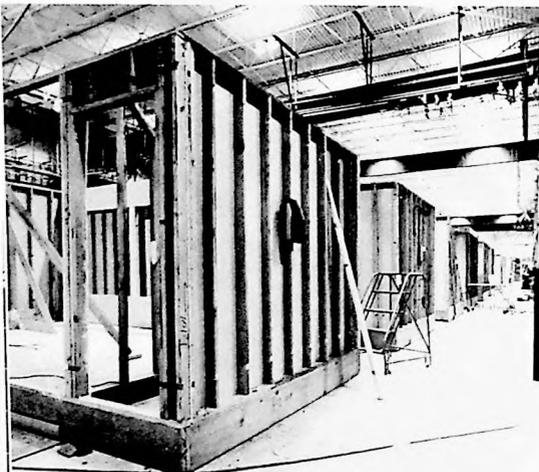
MODULE ON ASSEMBLY LINE AT LEVITT BATTLE CREEK PLANT
