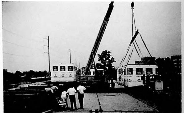
POSITION OF STRAPS JUST PRIOR TO CRANE TAKING UP SLACK ON GE MODULE BEING TRANSFERRED FROM HIGHWAY TRANSPORTER TO OTTX FLATCAR
