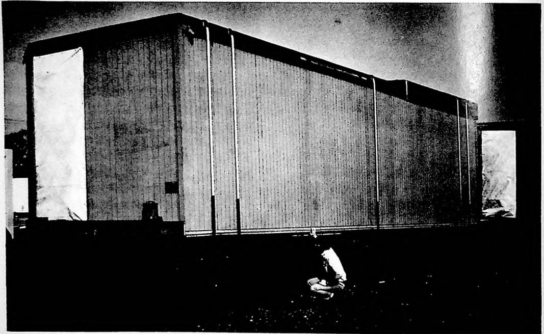
SECUREMENT OF MODULE TO TTCX FLATCAR BY VERTICAL DACRON STRAPS
