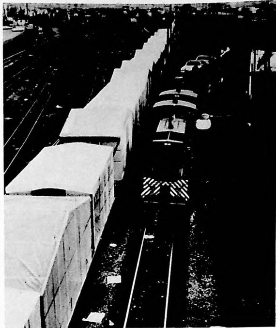
PHOTO DEPICTS A VERTICAL CLEARANCE POTENTIAL PROBLEM. COMPARE ROOF-PEAK HEIGHT TO THE ADJACENT TRI-LEVEL AUTO TRAINLOAD. MODULE'S SECUREMENT WAS INSTALLED TOO HIGH (ABOUT 4'-06") RESULTING IN ROOF HEIGHT OF 16'-06".
