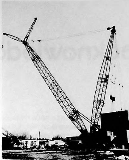
"SKY HORSE" CRANE, USED BY SHELLEY, TO HOIST AND POSITION CONCRETE MODULES AT JERSEY CITY.
