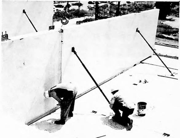
WALL-BRACING USED DURING ASSEMBLY OF DESCON'S UNITS
