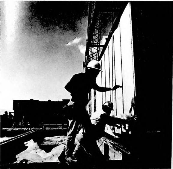
FINAL POSITIONING IS BY MANPOWER. NOTE PINCH BAR.
