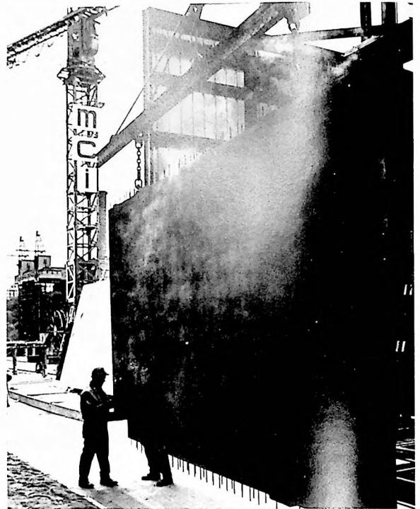
FLOOR PANEL BEING MOVED TO CURING AREA
