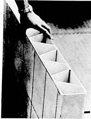
TYPICAL WALL CONSTRUCTION SHOWING CORRUGATED CORE AND SURFACE ELEMENTS
