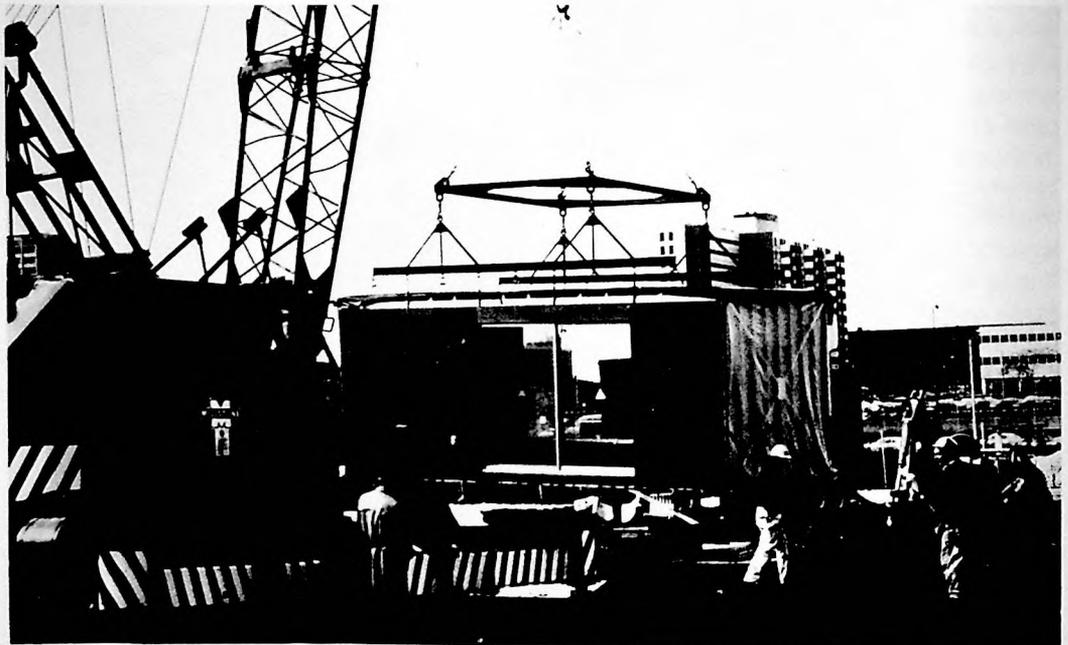
LIFTING FRAME BEING USED TO ERECT MODULES
