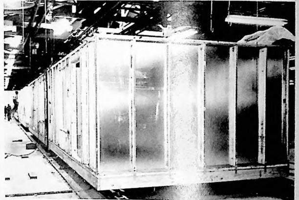
MODULE ASSEMBLY USING METAL STUDS
