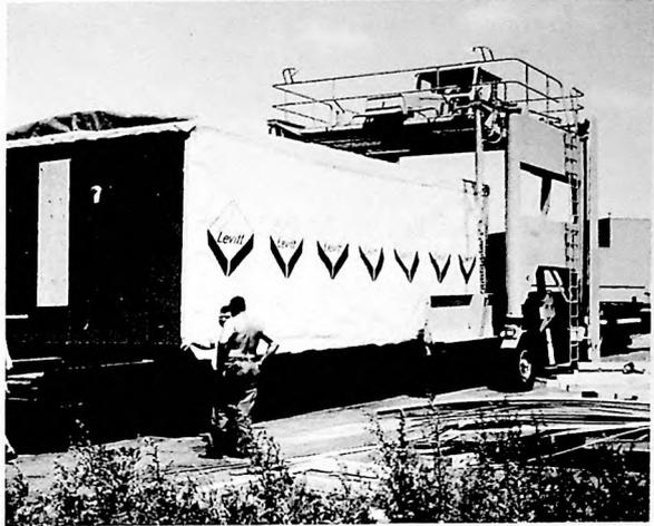
LEVITT PACKAGED MODULE BEING LOADED ON RAIL-CAR
