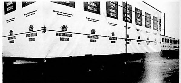
ORIGINAL PACKAGING THAT FAILED DURING FIRST RAIL SHIPMENT TO MEMPHIS AND WAS LATER REPLACED WITH CROSS-LAMINATED HIGH-DENSITY POLYETHYLENE
