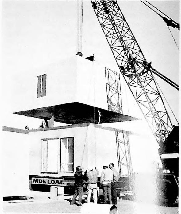
UPPER MODULE OF THE TWO-STORY UNIT BEING SET IN PLACE PRIOR TO SHIPMENT TO THE BUILDING SITE
