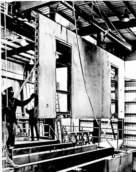
WALL PANEL BEING REMOVED FROM CASTING MOLD
