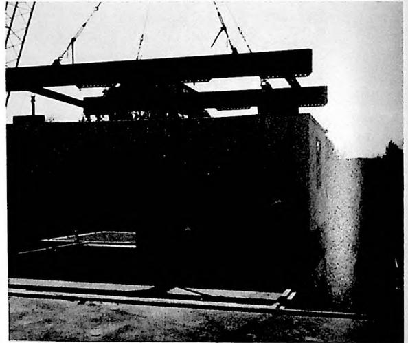
CTC SECOND-STORY MODULE BEING PLACED ON TOP OF FIRST-STORY MODULE (TWO MODULES ARE THEN PLACED ON TRANSPORTER AND MOVED AS A COMPLETE UNIT TO BUILDING SITE)
