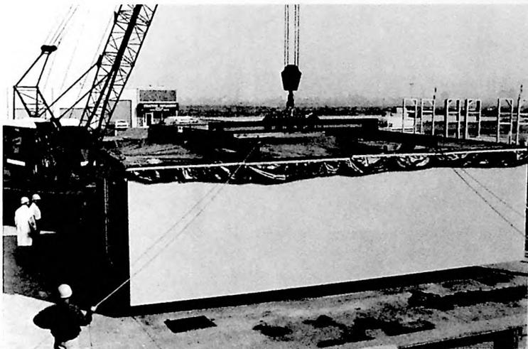
"H" SHAPED LIFTING FRAME USED TO LIFT SECOND STORY MODULES
