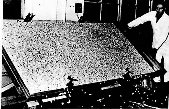
STRUCTURAL PANEL AFTER INCORPORATION OF STONE AGGREGATE
