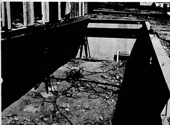
VIEW OF HOME FOUNDATION PRIOR TO TRANSVERSE POSITIONING OF SECOND HBC MODULE. NOTE HORIZONTAL TRANSFER BEAMS.
