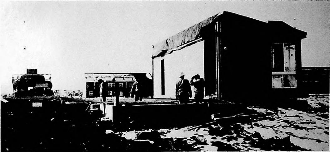
HBC PROTECTED MODULE IN PLACE AT SITE – PLYWOOD ON THE LEFT SIDE IS REMOVED PRIOR TO INSTALLATION OF ADJOINING MODULE
