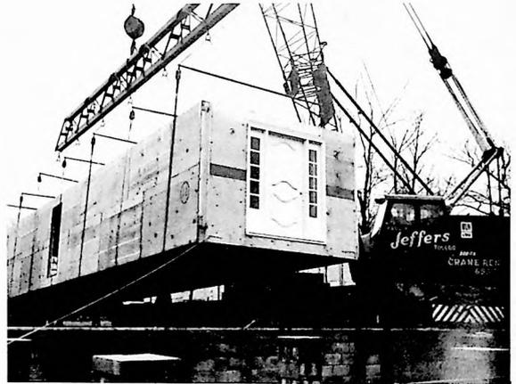
SCHOLZ MODULE BEING ERECTED AT INDIANAPOLIS — SHEATHED WALLS WERE USED TO PROVIDE ADDED STRENGTH
